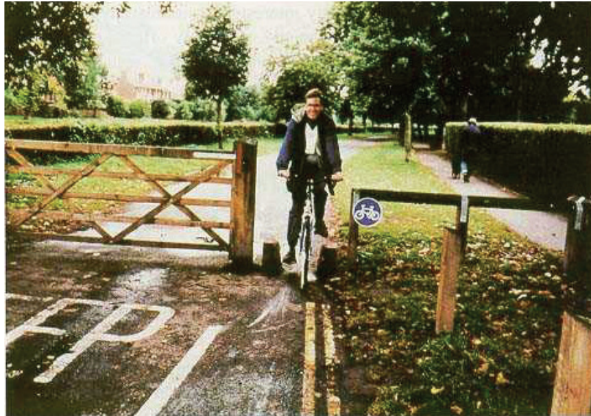
Figure 23-18. Photo. The entrance to this bicycle trail is designed to restrict entry to motor vehicles.
