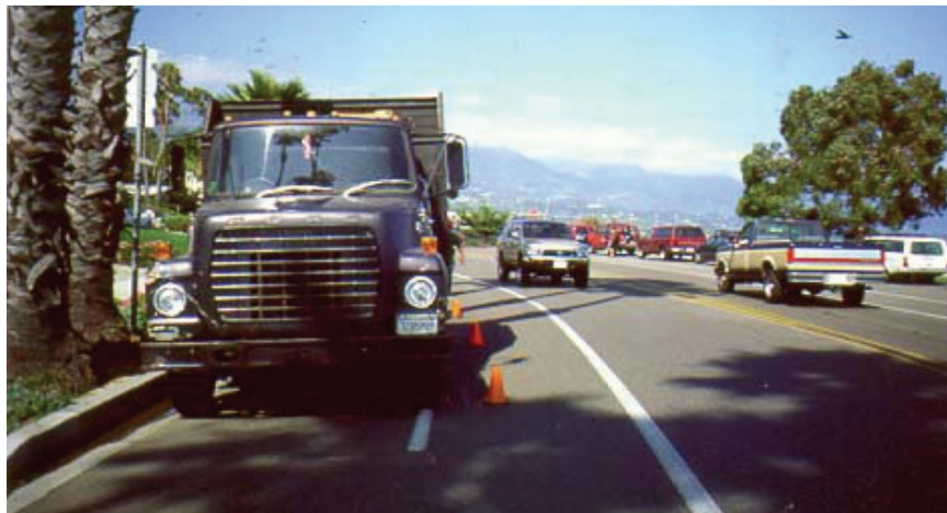
Figure 21-1. Photo. Utility work in bike lanes can often be accomplished without blocking the entire lane.
