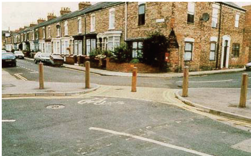
Figure 20-14. Photo. Diagonal road closures/diverters limit vehicular access but allow emergency vehicles to enter through removable bollards.
