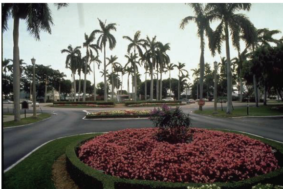
Figure 20-2. Photos. Traffic-calming devices are used to break up long, uninterrupted street vistas that encourage speeding.
