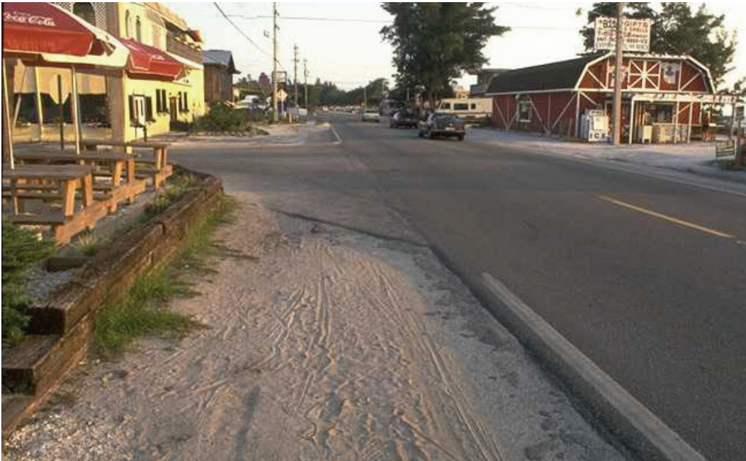
Figure 16-2. Photo. Roadways with paved shoulders should reduce on-road debris.
