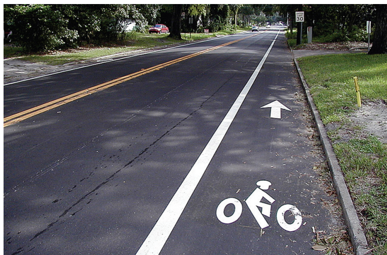
Figure 16-4. Photo. Example of newly striped bicycle lane with accumulation of debris next to curb.
