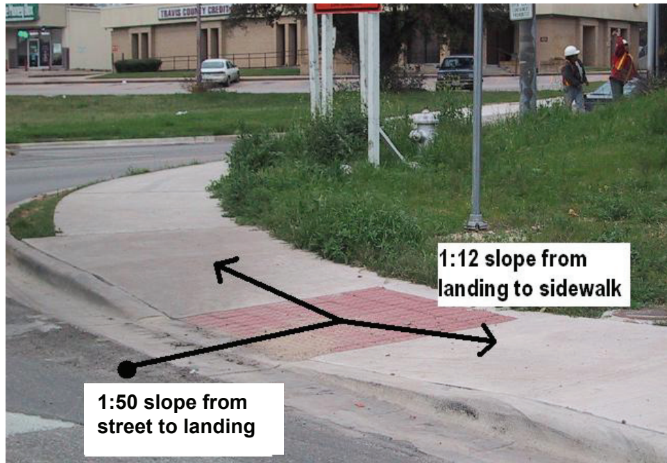
Figure 8-16. Photo. Parallel curb ramp.
