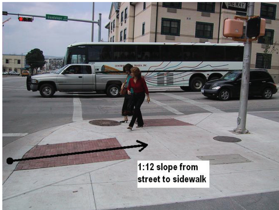
Figure 8-15. Photo. Perpendicular curb ramp.
