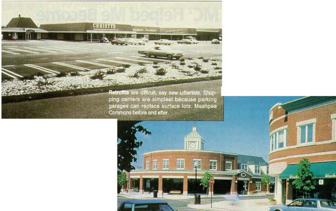
Figure 6-2. Photos. Mashpee Commons before and after retrofitting.
