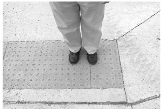
To enhance safety for people who are visually impaired, ADA accessibility guidelines require that truncated dome surfaces, like the one shown here, be installed on new curb ramps and any alterations to existing ramps.
