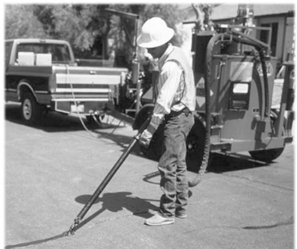
A worker is shown sealing a pavement crack. Crack sealing is one of a variety of cost-effective, thin-surface treatments that can help preserve and extend the service life of pavement.
