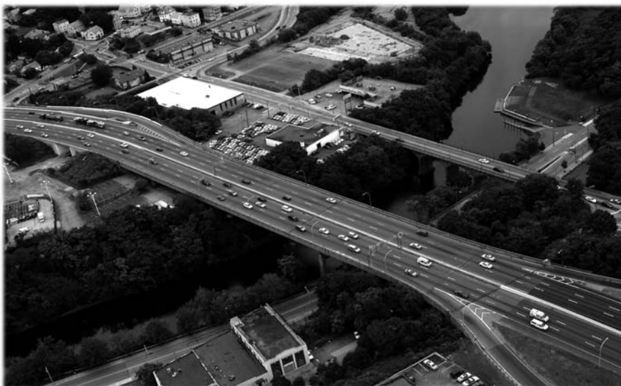
Bridge No. 550 in Pawtucket, RI, is a badly deteriorated structure that is part of the busy I-95 north-south corridor. The bridge carries an average daily traffic load of 175,000 vehicles.
