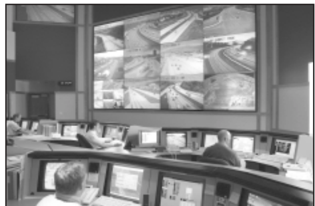
The control room for Utah DOT's test project includes screens displaying weather and road conditions and traffic information.
