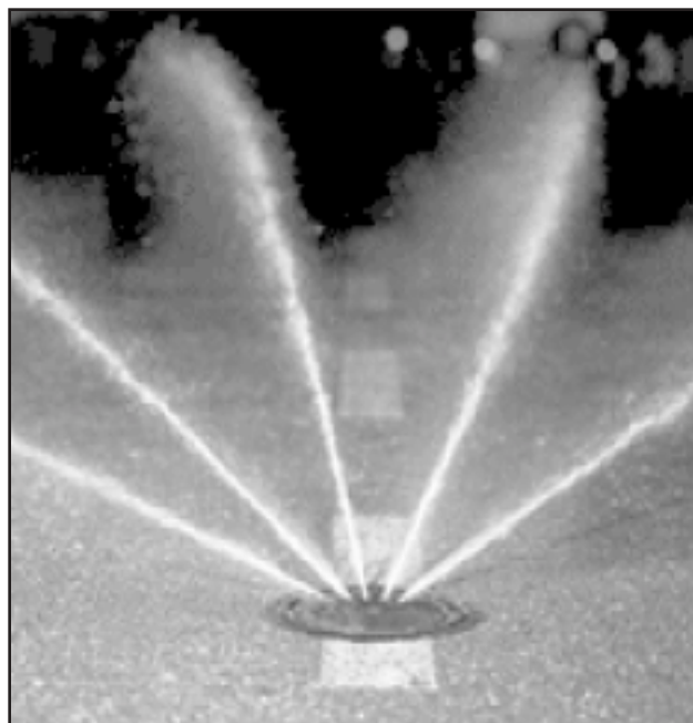
Fixed anti-icing systems, such as the system shown here, use sensors to predict the freezing point of the road surface and activate the anti-icing spray system.
