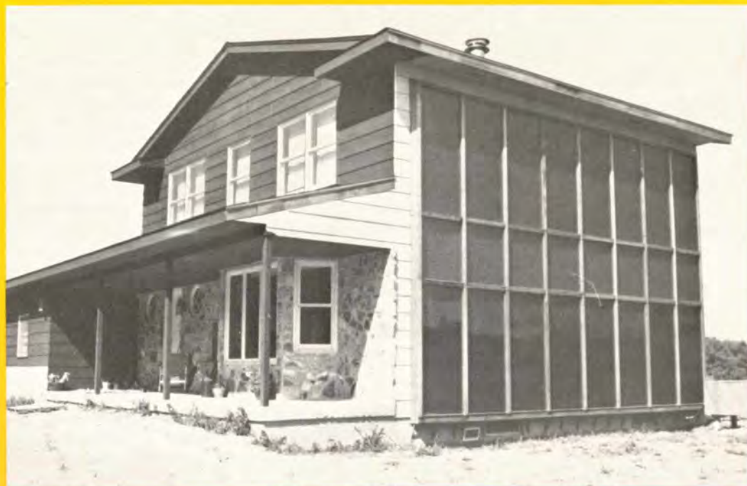
A conventional-looking house except for the south-facing window wall, which isn't a window at all. It's a passive solar collector for hot water and space heating.
