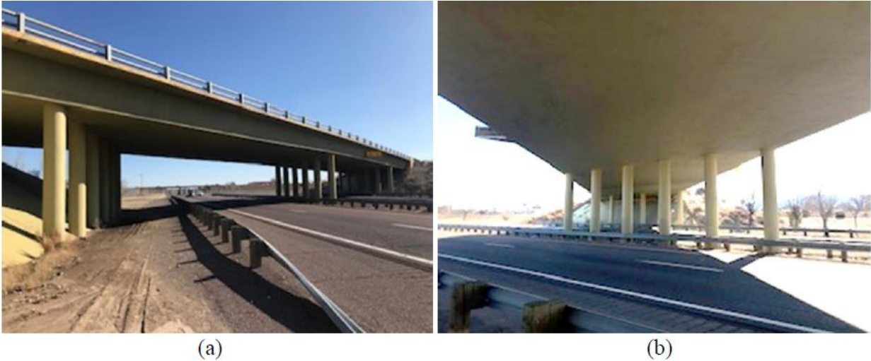
Figure 6.25. Bridge No. 7032 - a) plan view; b) bottom of multicell box girder superstructure; (UHPC Phase V, Figure 5.1)
