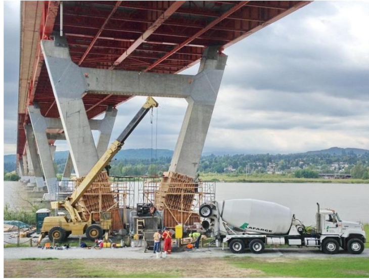
Figure 7.5. Casting of UHPC Jacquet of Pier S4
