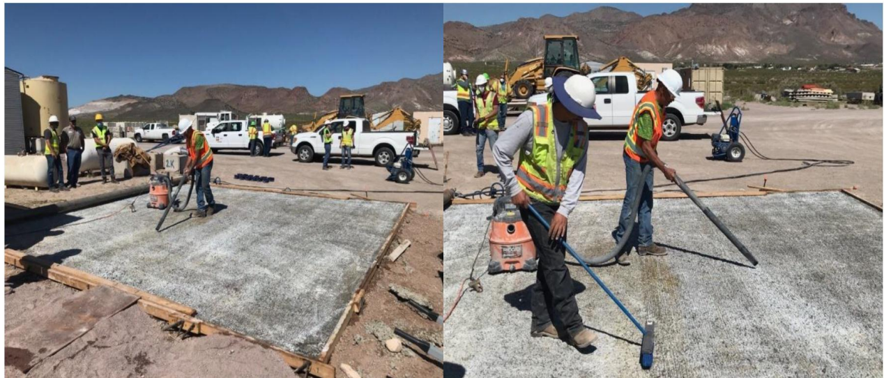
Figure 6.21. HPD surface preparation (UHPC Phase V, Figure 4.1)
