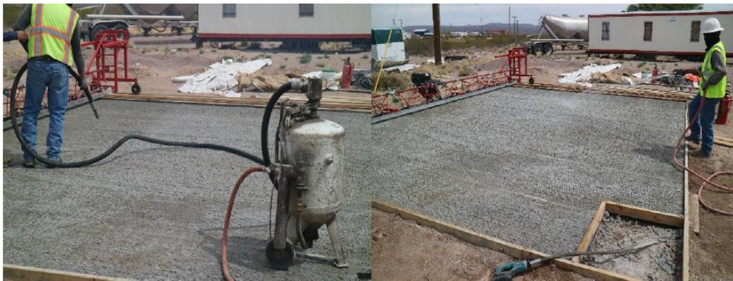
Figure 6.24. Mock up No. 4 - HPD surface preparation (UHPC Phase V, Figure 4.11)
