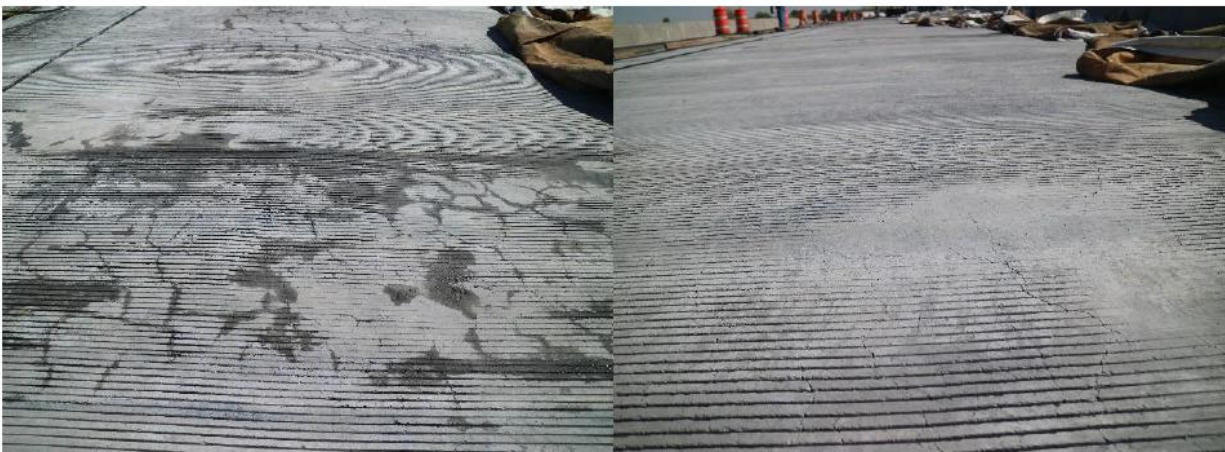
Figure 6.27. Overlay cracking from production placement 1 (UHPC Phase V, Figure 5.9)
