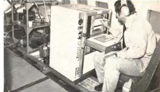
John Morrow checks a data recorder aboard an FAA Boeing 727 flying a Small Community MLS demo at Shiraz, Iran.
