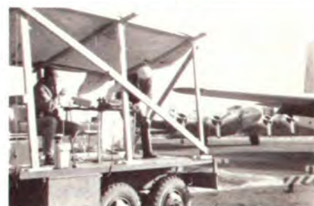
Reno, Nev., controllers at the Chester, Calif., Airport were cheek-by-jowl with the fire bombers in their temporary tower aboard a Forest Service flat-bed truck.
