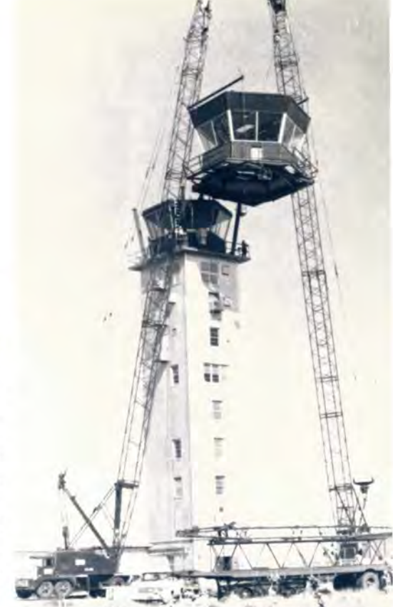
The Albuquerque, N.M., tower got a crown upon its crown during a modernization designed to increase its height and space for more modern equipment. The old cab is now used for a training facility.
