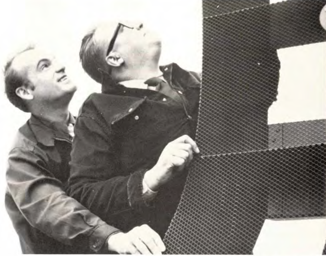
Technicians Paul Seewerker (left) and John Kubiak guide the ASR-8 antenna sail as a crane starts lifting it to the top of a 75-foot tower.
