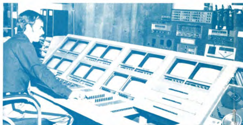
14 EYES PLUS 2 —An Aeronautical Center security officer checks the monitors at the Security Control Center, part of a system of closed-circuit TV spotted around the Oklahoma facility. It includes two-way communications for identification of off-hours visitors and unlocking of entrance doors by the officer via an electric switch.
