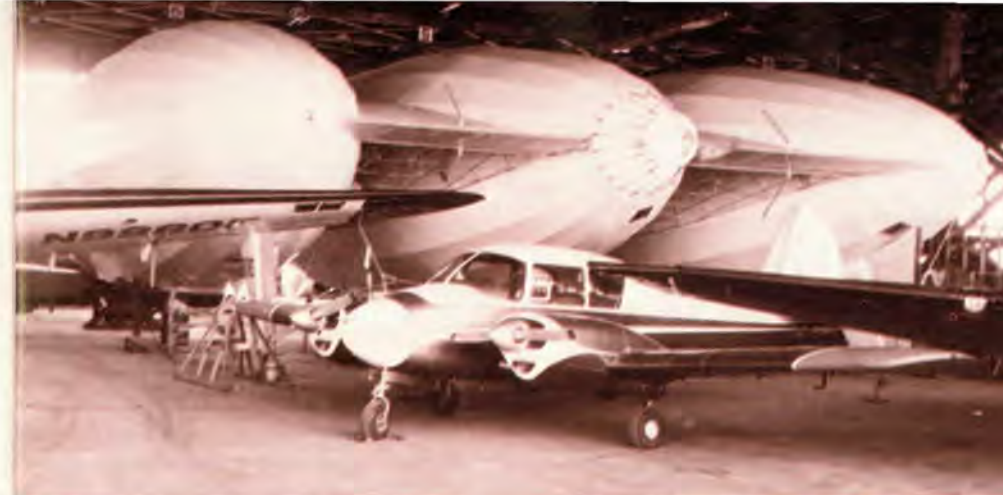
The triple-hulled Aeron III was built in the hangar at Mercer County Airport in Trenton, N.J. Damaged during taxi tests, it never did get off the ground.
