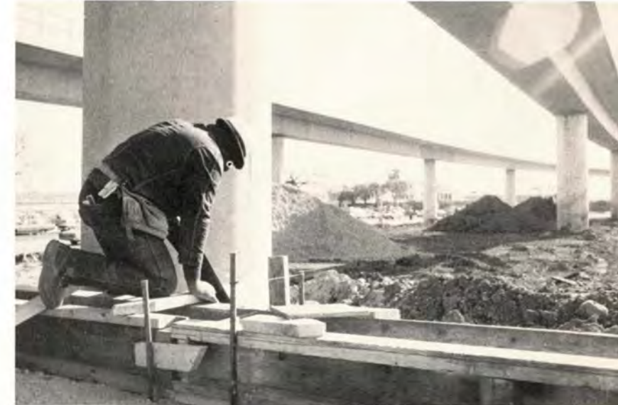
A Metro worker builds a concrete form at the base of the railway's pillared superstructure. The main terminal and airport control tower can be seen in the distance.
