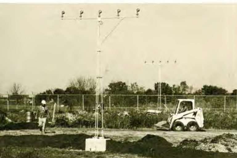
New frangible approach light systems were installed at O'Hare last year. If accidentally struck by aircraft, the lights will break away with minimal aircraft damage.
