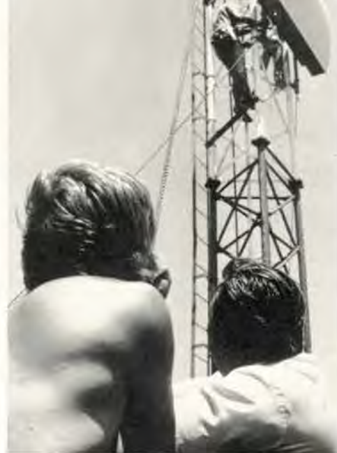
Airway Facilities technicians raise a portion of a glide-slope antenna at O'Hare International Airport. Solid-state glide slopes were among the new instrument landing system components installed at airports in the Great Lakes Region this past summer.
