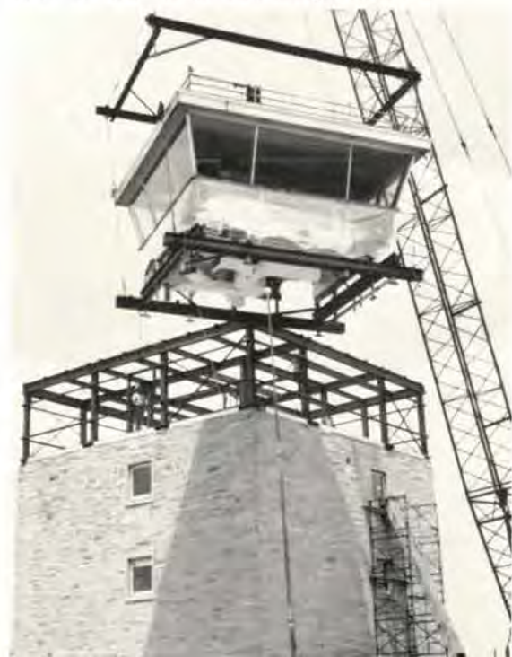
The 25-ton tower cab at the University of Illinois-Willard Airport was removed to make way for a one-story addition, then replaced and operated while the floor below was being completed.
