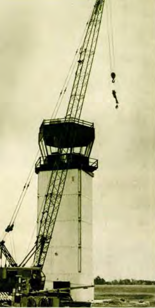
The cab of this new modular tower at the Johnson County, Kan., Airport was set in place in 25 minutes—in record time—last August.
