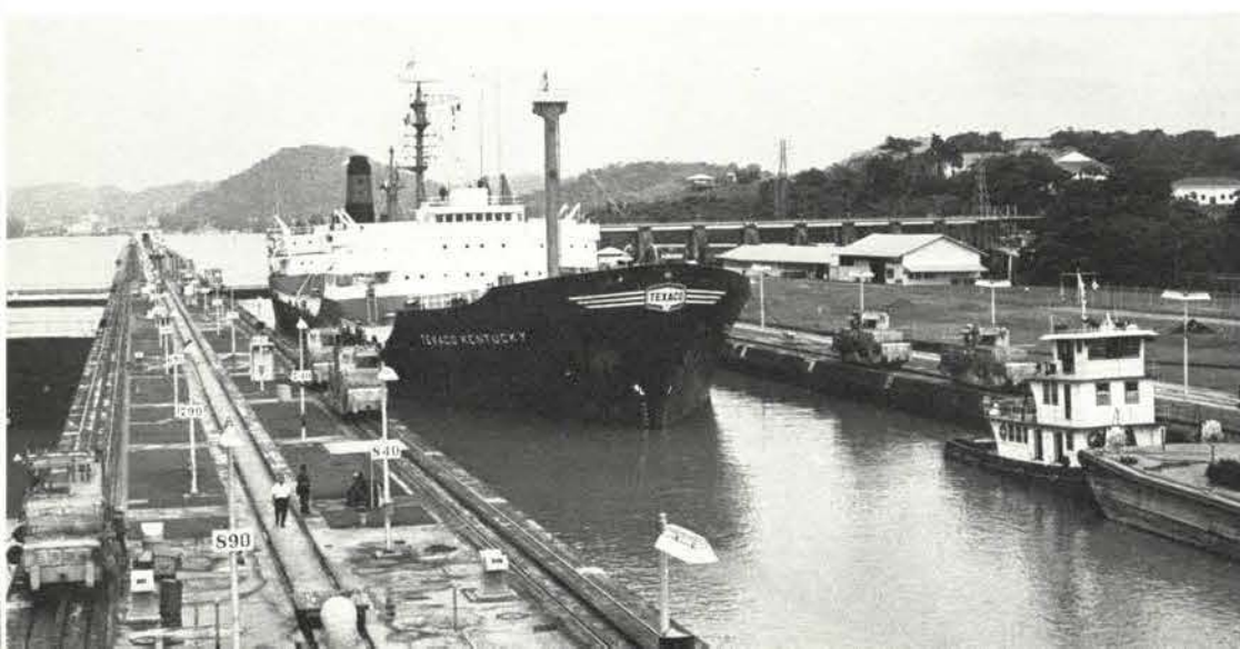
A tanker moves through the mile-long Miraflores Locks en route from the Atlantic to the Pacific. These locks raise or lower ships in two steps a total of 54 feet.
