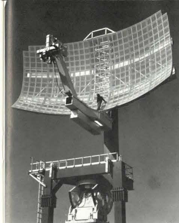
POWERFUL EYE —FAA has contracted for 16 advanced Air Route Surveillance Radars (ARSR-3) to serve high-density air-traffic areas. They will provide improved target and weather detection and reduced clutter. The first—to be delivered in two years—will go to the Aeronautical Center for training purposes.
