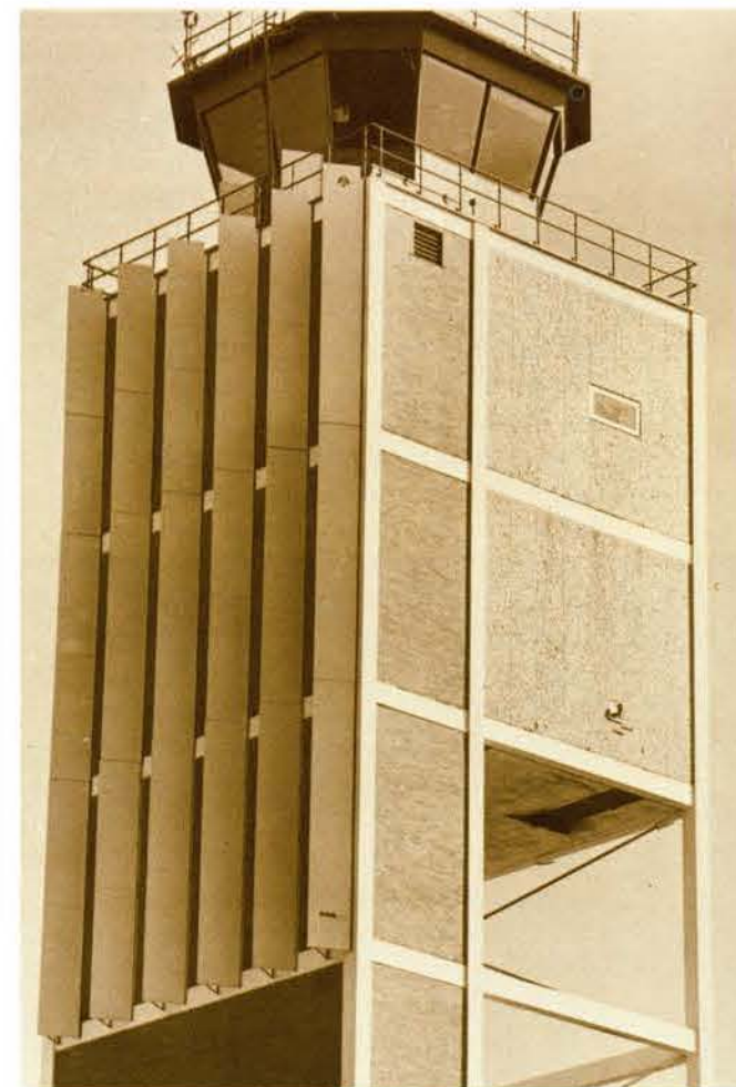
GHOST BREAKER —The Tulsa, Okla., Tower was the test bed for an electromagnetic energy absorbing material developed by Rockwell International for eliminating ghost images on airport radar tracking scopes. In this case, the tower wall was the reflecting culprit, and installation of the absorptive panels turned the trick. Rockwell International Photo
