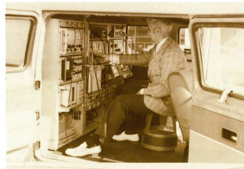
INTERFERENCE BAN VAN —Increasing congestion of radio frequencies has resulted in greater interference with aviation frequencies from such things as plastic welders, ships, garage-door openers, cars and other radio stations. To the rescue is this self-contained Electromagnetic Interference Van, which detects and measures the interference. John Guest, frequency manager of the Central Region operates the van.
