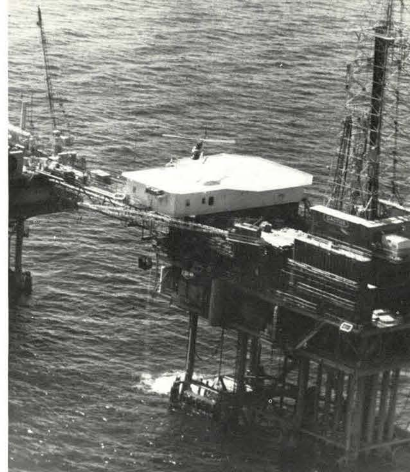
Alighting on an oil-drilling-rig helipad is a Bell 206B Jet Ranger, some 110 miles off Intracoastal City, La. At left, connected by bridgework is a production rig, which connects to shore refineries via a pipeline.
