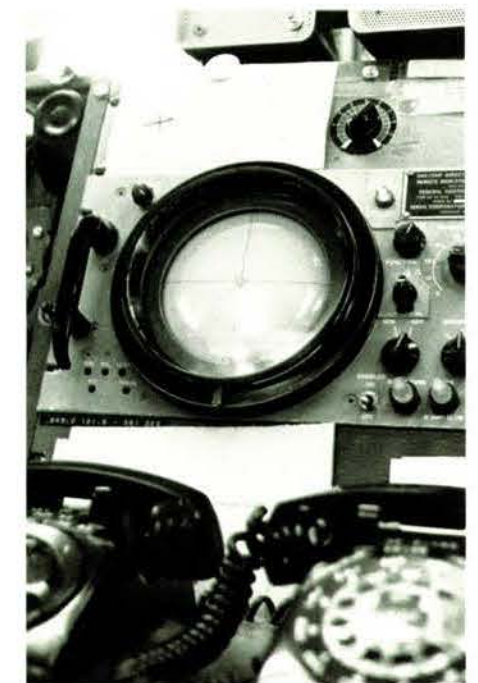
Pilots' lives depend on this small circular scope — Martinsburg's radio direction-finding console, which is effective to 100 miles, but usually gets closer work. The DF antenna is on the opposite page.
