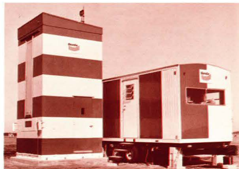
Another glide-slope antenna and equipment shelter provides a signal for flare out and touch down on instruments.
