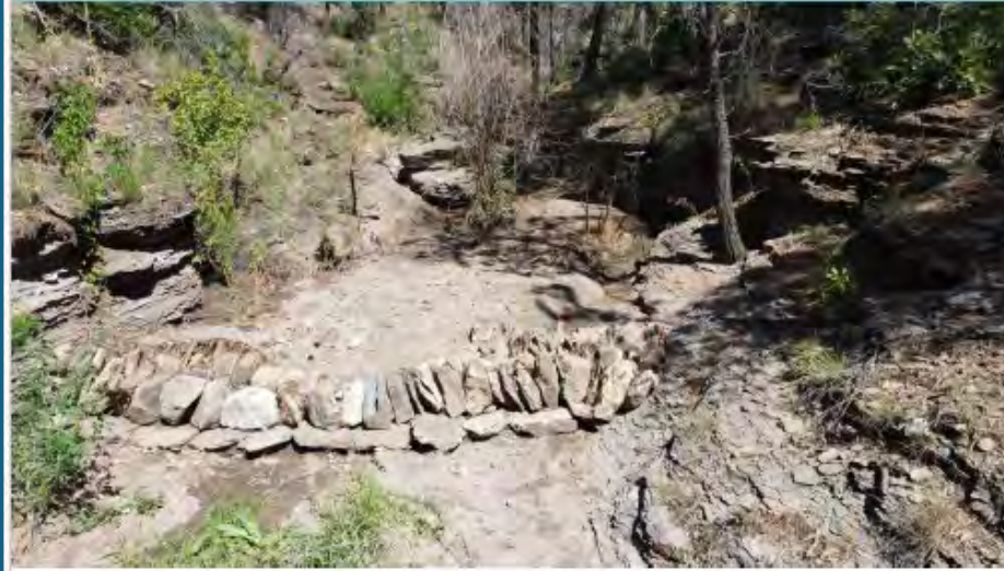
One Rock Dam constructed by HPWA seasonal crews in Gallinas (Summer 2023).
