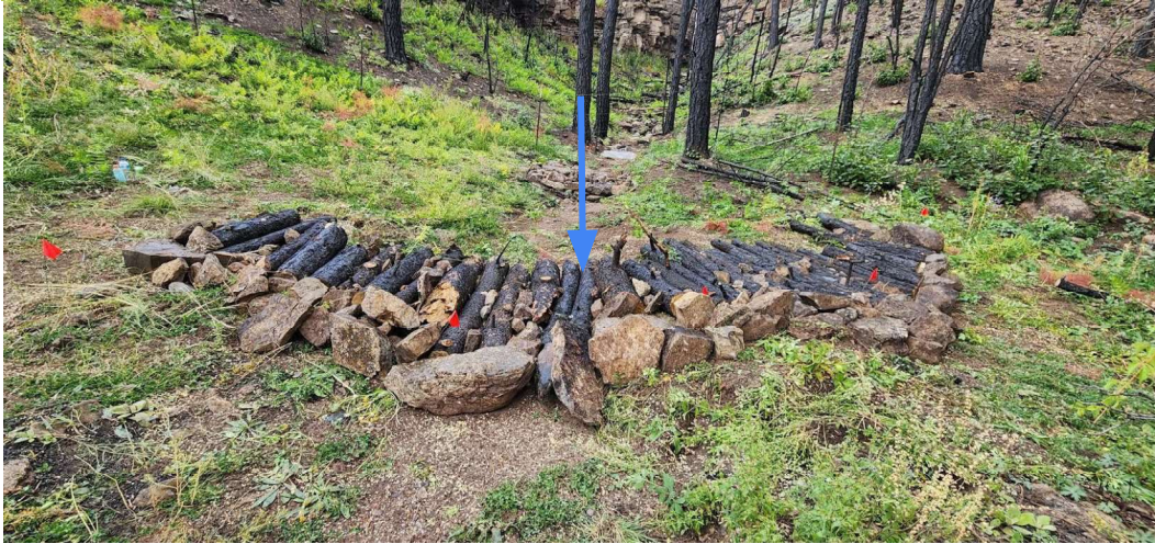
Media Luna constructed of logs by HPWA seasonal crews (Summer 2023).
