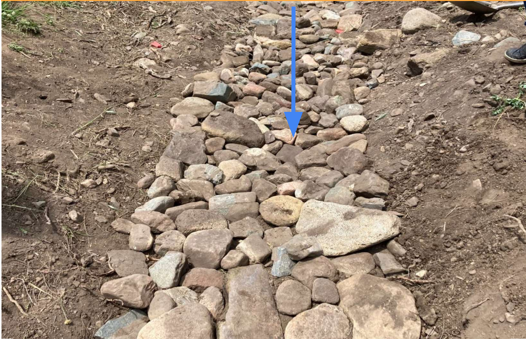
Rock Rundown constructed by HPWA seasonal crews in Sapello (Summer 2023).
