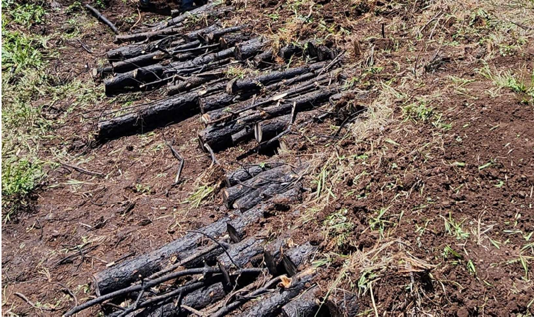
Log Mat to stabilize a channel side slope constructed by HPWA seasonal crews (Summer 2023).
