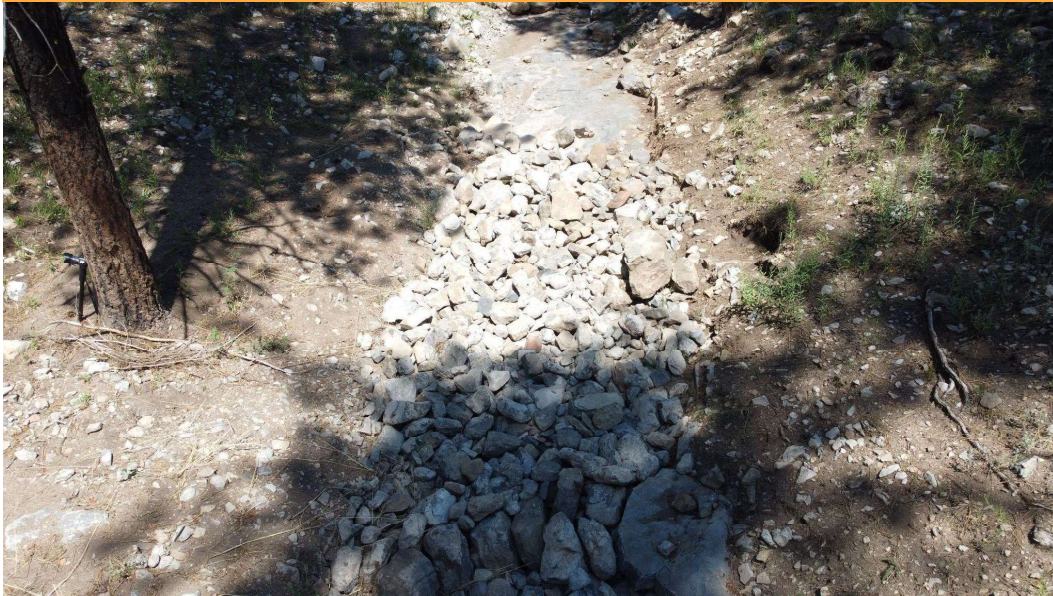
Rock Rundown constructed by HPWA seasonal crew in Sapello (Summer 2023).
