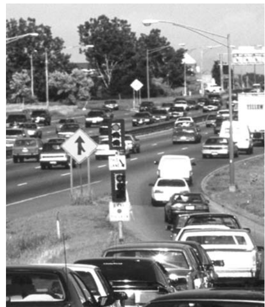
Ramp metering systems, such as the one shown here, are one example of the type of ITS projects described in FHWA's new ITS online reference tools.
