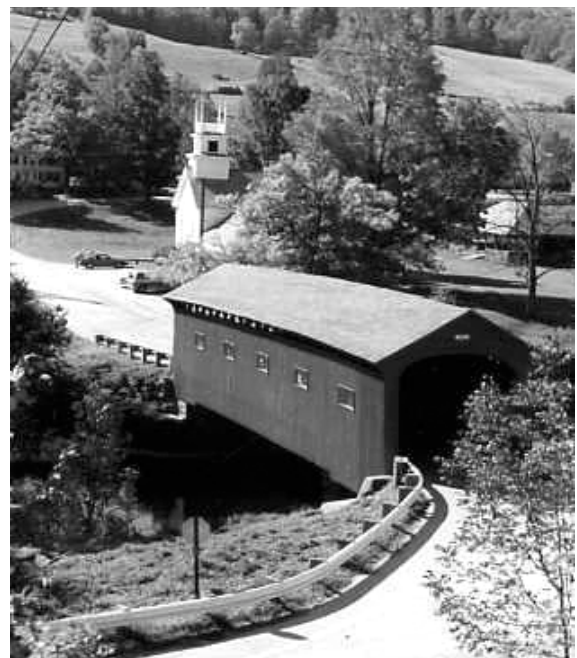
On July 21, 2004, FHWA will hold a seminar on covered bridges like this one. The seminar will coincide with the release of the Covered Bridge Manual .
