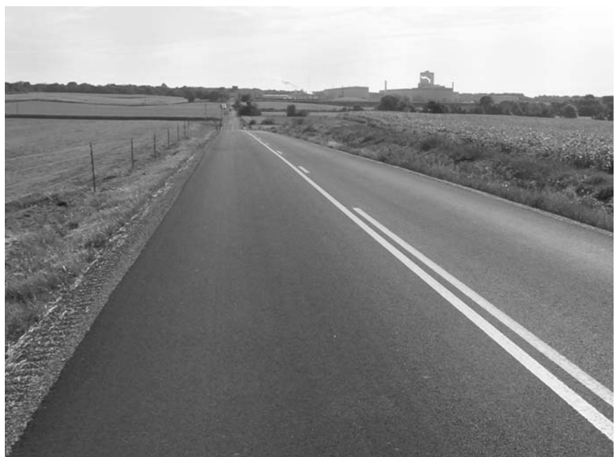
This section of highway in Indiana features asphalt pavement designed using Superpave.
