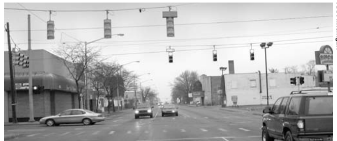
After the RSA, three traffic signal heads were suspended on a box span of wire directly over the travel lanes, with two signals for the through lane and one for the left turn lane. Traffic signal timing also was adjusted to add a protected left-turn phase. In addition, pavement markings now show a separate left-turn lane at the intersection.
