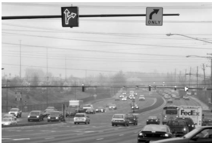
FHWA's new guide on signalized intersections includes information on ways to improve traffic flow at busy intersections, such as the one shown above.
