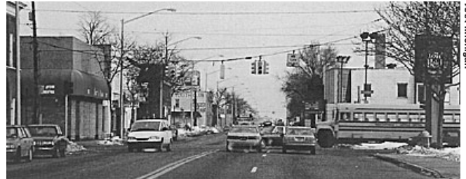
Prior to the RSA of this intersection in Grand Rapids, MI, two traffic signal heads were suspended on a diagonal span of wire with only one head hung over the travel lanes. The intersection also had two approaching lanes, which were separated by a dashed white pavement marking.
