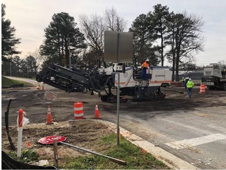
Figure 10. Asphalt Surface Milling in Preparation for Slab Placement
