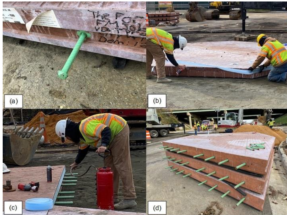
Figure 14. Panel Installation Details for Laburnum Avenue: (a) Screw-in Tie Bar; (b) Blue Polyethylene Ribbon and Joint Filler; (c) Bond-Breaking Oil Spraying; (d) Foam Gasket to Prevent Grout Leak
