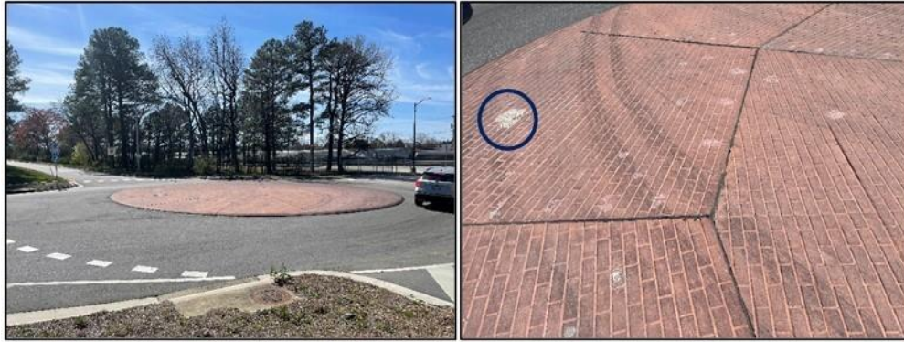
Figure 28. Surface Condition of Laburnum Avenue Precast Mini-Roundabout in 2023
