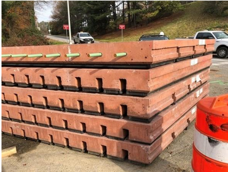
Figure 11. Precast Slabs Stored on Site before Construction
