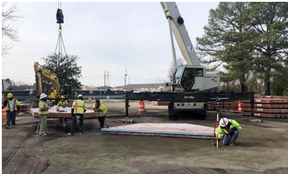
Figure 13. Installing the Center Panel and Surveying to Set Proper Grade
