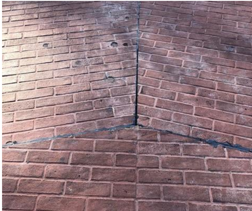
Figure 17. Joint Sealing with Silicon Sealer
