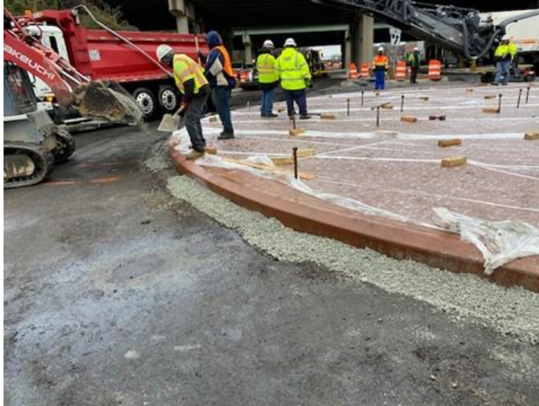
Figure 20. Dense-Graded Base Aggregate Placed around the Perimeter to Prevent Grout Leakage
