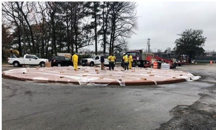
Figure 15. Panels Covered with Plastic Sheetting to Prevent Rain Damage
