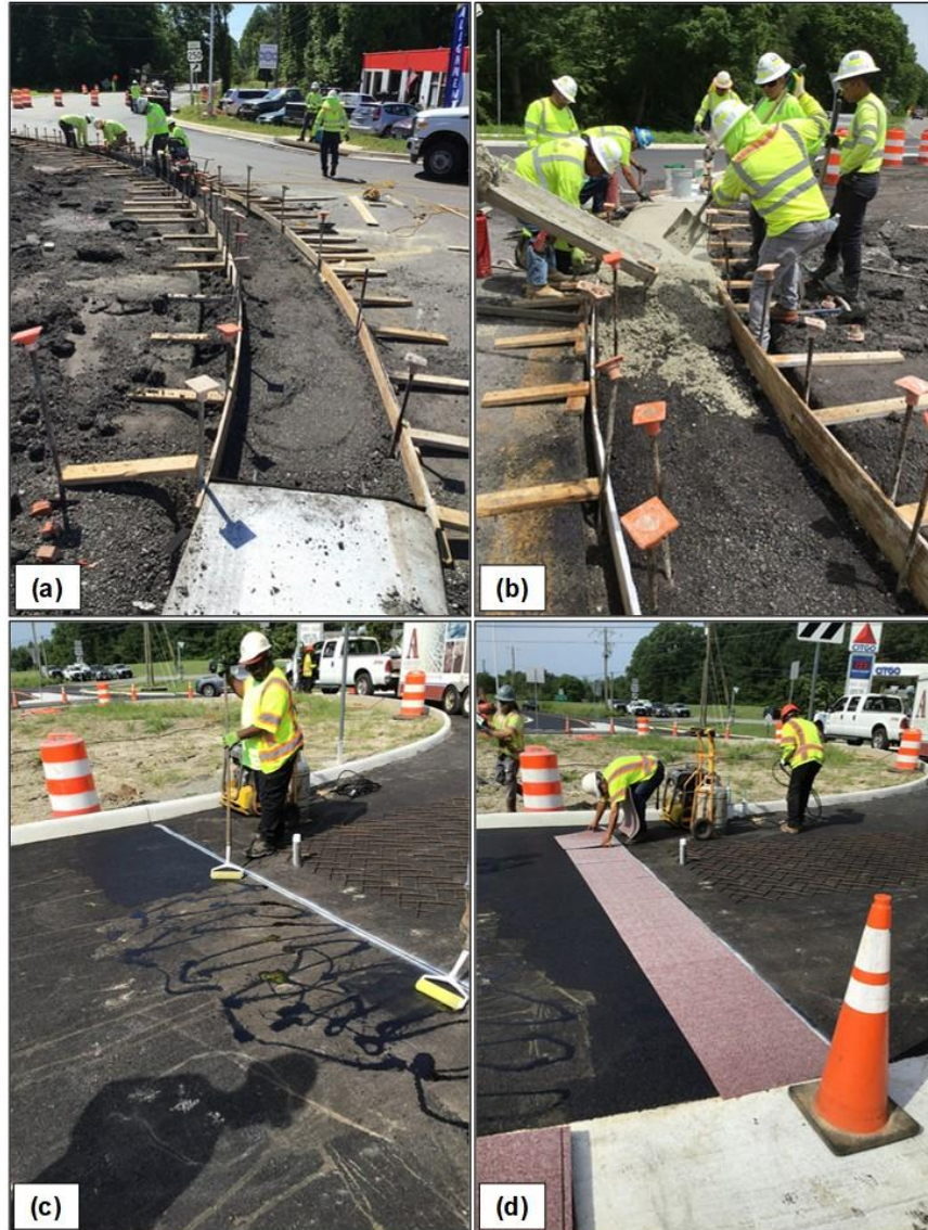
Figure 26. Gum Spring Roundabout Construction: (a) Form Work for the Outer Curb; (b) Concrete with Rapid-Setting Cement in the Curb; (c) Glue Application on the Asphalt Truck Apron; (d) Installation of Red Thermoplastic Sheets (Courtesy of VDOT's Culpeper District)
