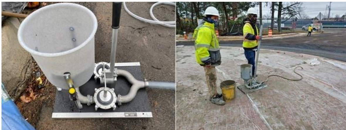
Figure 19. Grouting Operation Using a Hand Pump
