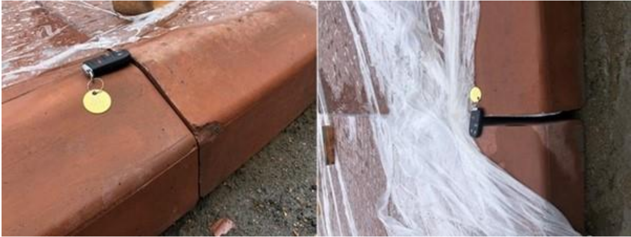
Figure 16. Panel Fitting with Minor Gaps at Laburnum Avenue Precast
