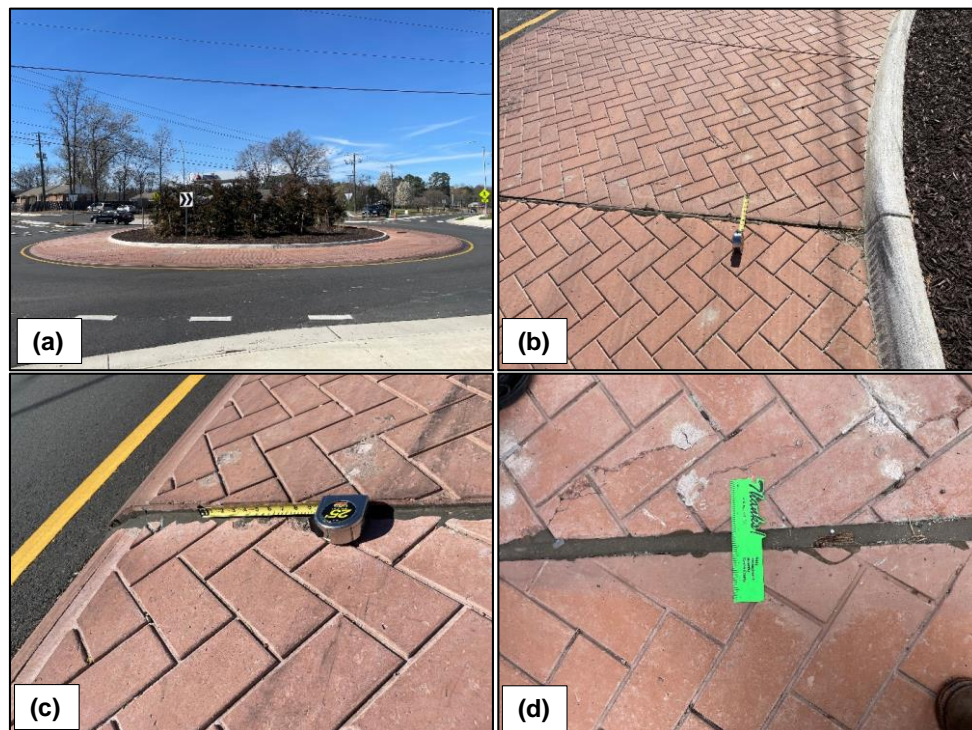
Figure 29. Hopkins Road Precast Roundabout Surface Condition in 2023: (a) Completed Truck Apron; (b) Ground Panel to Match Elevation; (c) Panel Drop-off in One Location; (d) A Few Cracks Near a Joint
