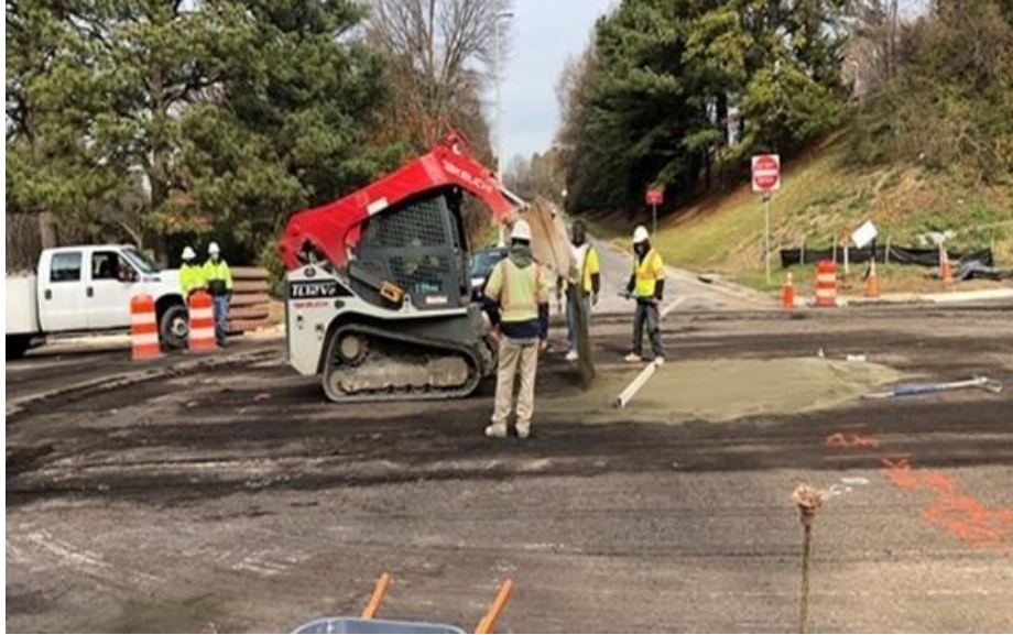
Figure 12. Using a Sand-Cement Mixture to Achieve Final Grade before Panel Installation
