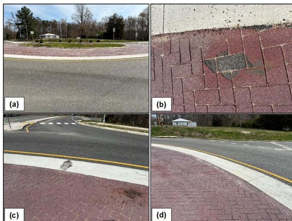
Figure 31. Gum Spring Roundabout Surface Condition in 2024: (a) Seemingly Accidental Damage to Roundabout; (b) Thermoplastic Surface Worn off; (c) One Crack on Rapid-Setting Cement Concrete Curb; (d) Some Settlement at the Thermoplastic Edge
