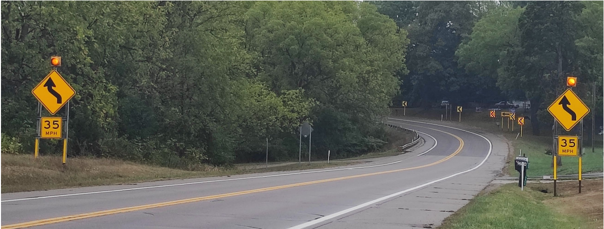
Figure 31. Example of Flashing LED Chevrons (background) and Flashing Warning Beacons (foreground) at WB US-12 Person Highway (Site 3)
