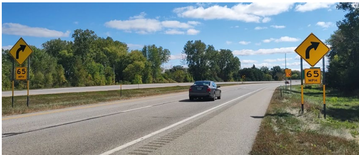
Figure 20. Example DSFS Message Display at Freeway Mainline Curve Site 1
