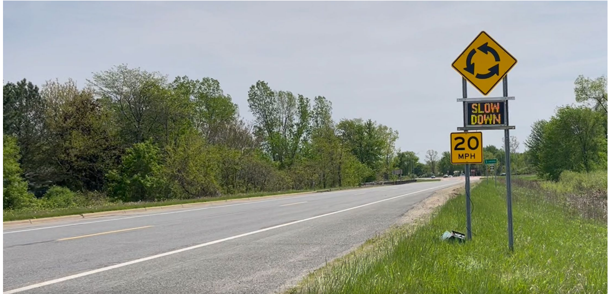
Figure 59. Example DSFS Message Display (Site 2, EB M-43 Grand Ledge)
