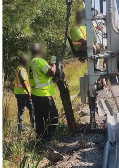
(b) Pulling out damaged posts.
