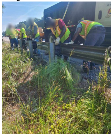
(e) Installing guardrail sections and tightening all bolts
