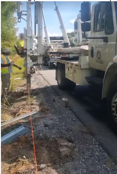
(c) Setting up a stringline to position posts at the proper alignment, and spacing
