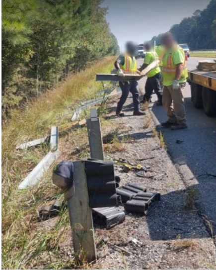
(a) Removing parts that cannot be repaired
