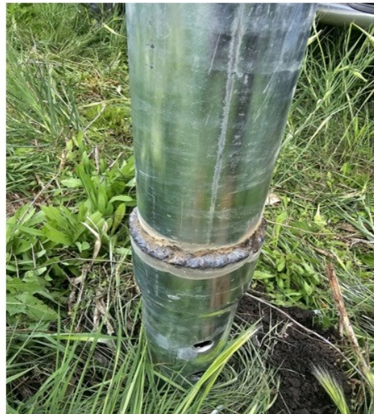
(d) Welded connection to connect helical pile with the above ground post
