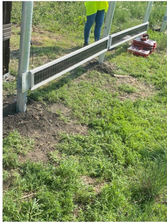
(b) View of strips of solar snow fence
