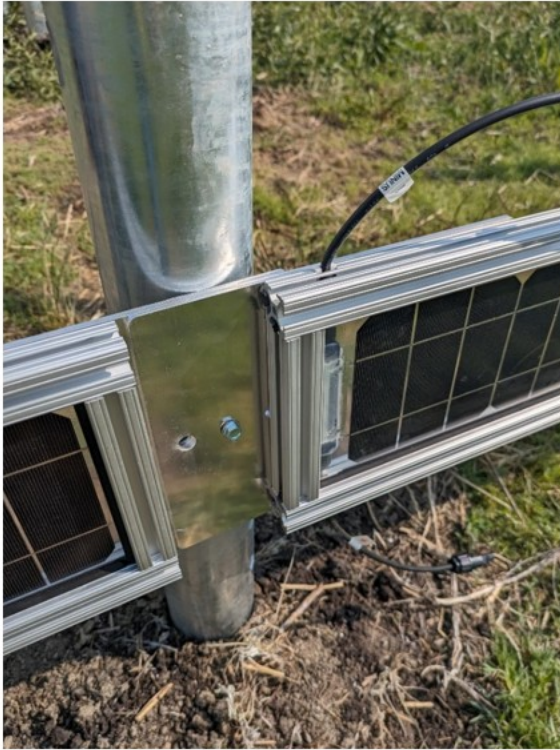
(a) Connection of solar panels onto posts
