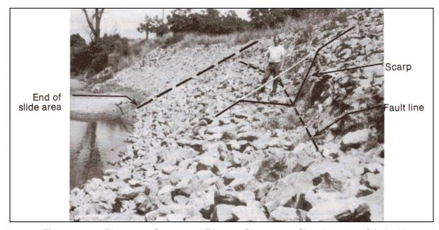
Figure 5.11. Riprap on Cosumnes River at Site 2 near Sloughhouse, CA, looking downstream, showing translational slide failure (photographed May 31, 1983) (Blodgett & McConaughy 1986).
