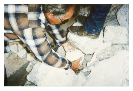
Figure 9.32. Installation of a float out device by Nevada DOT to monitor riprap stability.
