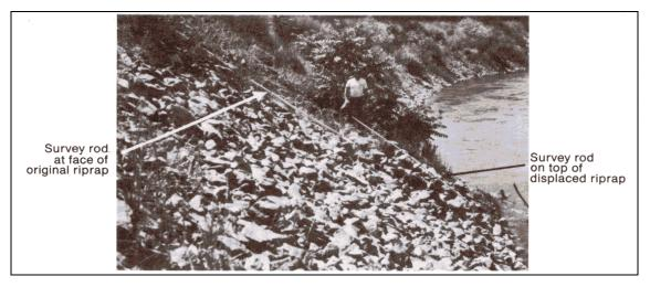
Figure 5.13. Riprap on Consumnes River at Site 3 near Sloughhouse, CA, looking downstream, showing modified slump failure (photographed May 31, 1983) (Blodgett & McConaughy 1986).
