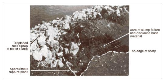
Figure 5.15. Riprap on left bank Cosumnes River at Site 1 near Sloughhouse, CA, showing slump failure (photographed May 31, 1983) (Blodgett & McConaughy 1986).
