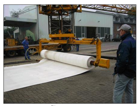
Figure 5.3. SandMat<sup>™</sup> geocomposite blanket being unrolled. (photo from NCHRP Project 24-07(2), courtesy Colcrete – Von Essen Inc.)
