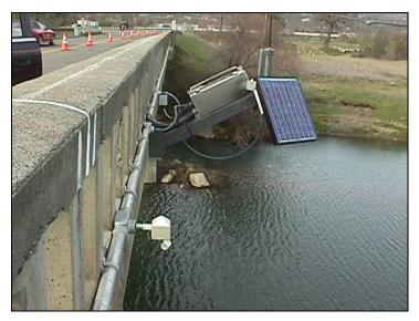
Figure 9.18. Tilt meter on California bridge.
