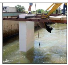
Placing geotextile containers with small front-end loader into scour hole at pier
