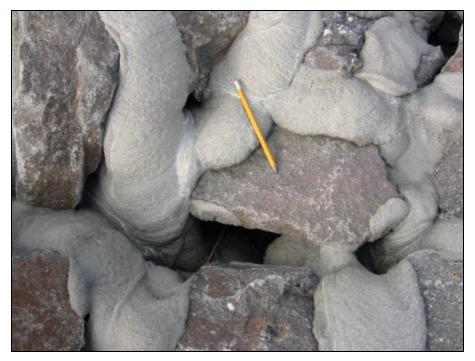
Figure 5.20. Close-up view of partially grouted riprap.
