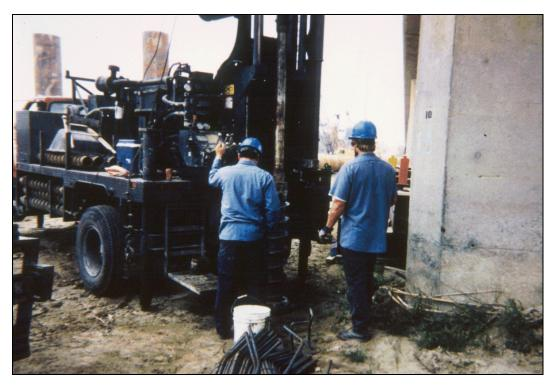
Figure 9.29. CALTRANS drilling with hollow stem auger for installation of float out devices at Salinas River Bridge (Highway 101) near Soledad, CA.
