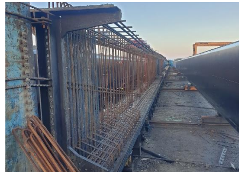
(d-1) Rebar caging for Tx-62
