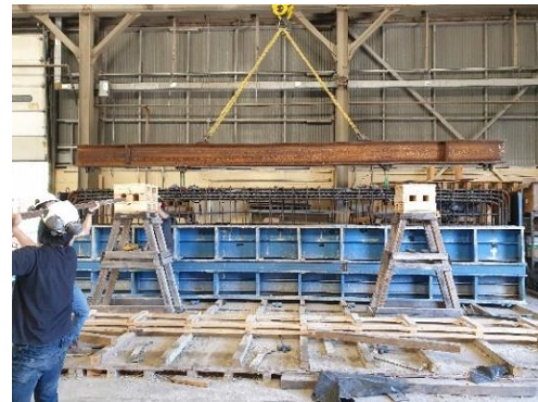
(b) Assembly of steel formwork
