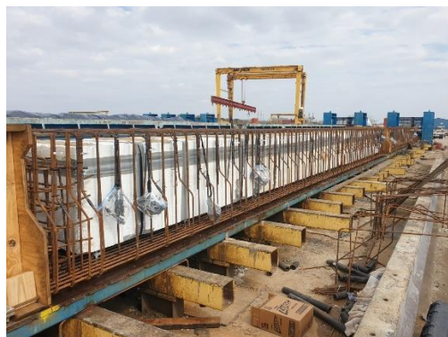
(d-2) Rebar caging for 5B40
