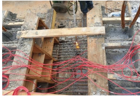
(h) Prestress releasing
