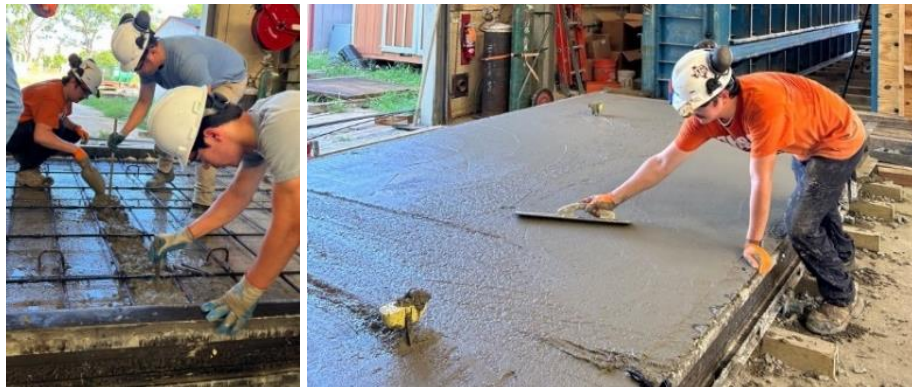
(c) Concrete casting
