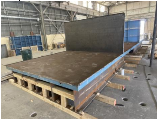
(a) Steel formwork and supporting frame
