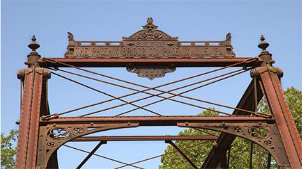
Figure B12. Botetourt County Structure No. 6386: Closeup of Portal (Before Painting) Showing Details of Phoenix Columns and Iron Decorative Elements
