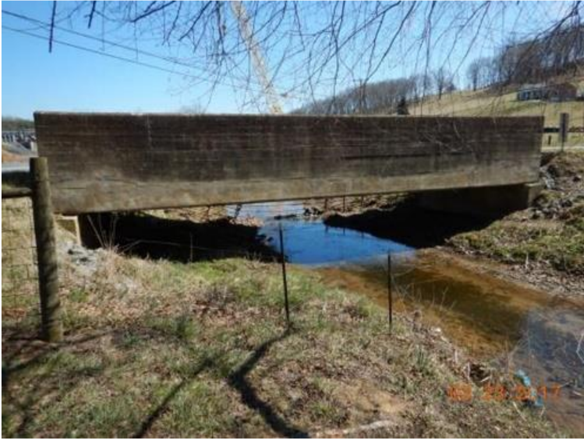
Figure B4. Another View of Augusta County Structure No. 6113, Showing the Typical Heavy Parapets of an Early Through-Girder Concrete Bridge
