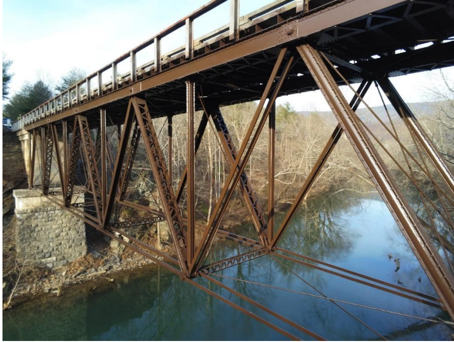
Figure B11. Botetourt County Structure No. 6100, Showing Phoenix Column Compression Members
