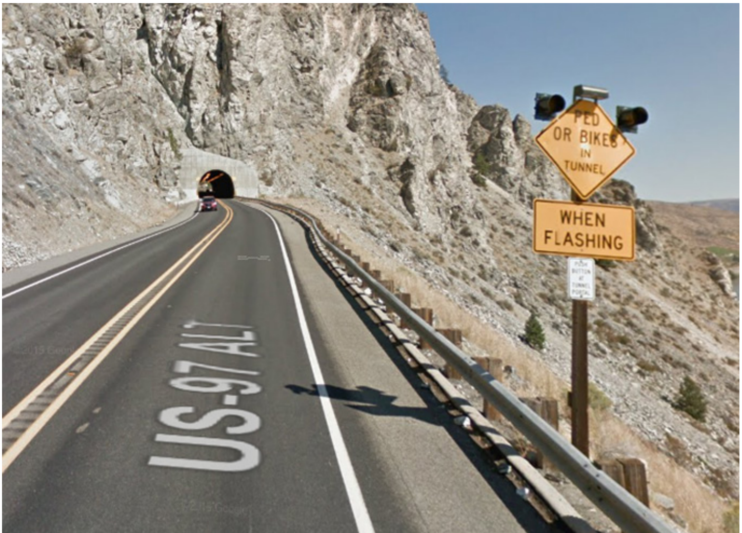
Figure 4-15: Bicyclist-activated dynamic warning beacons indicate to vehicles that bicyclists are present on the road. (Source: Google Streetview)
