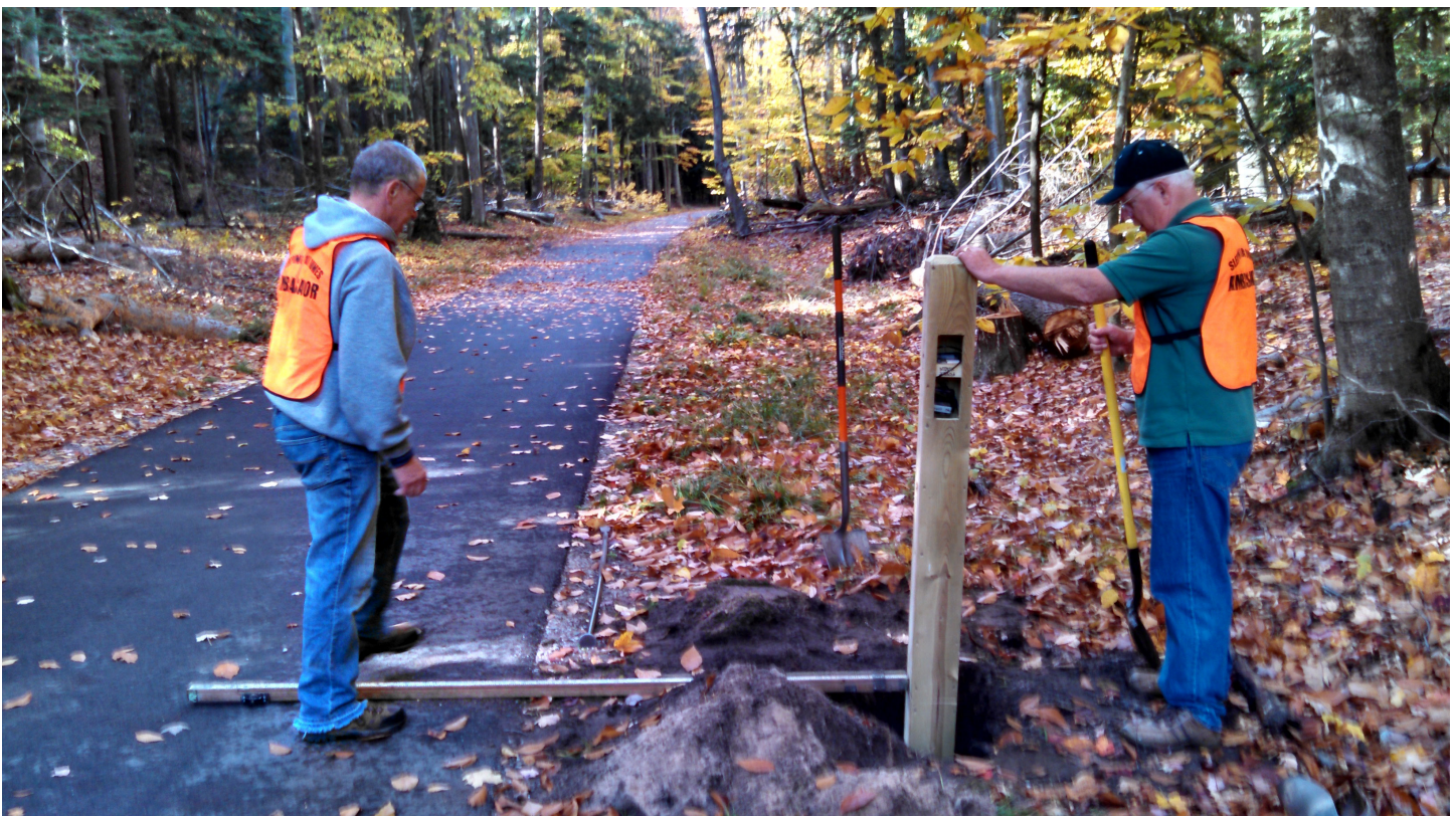
Figure 10-2: Installation of a pedestrian counter at Sleeping Bear Dunes National Lakeshore in Michigan. (Source: NPS)
