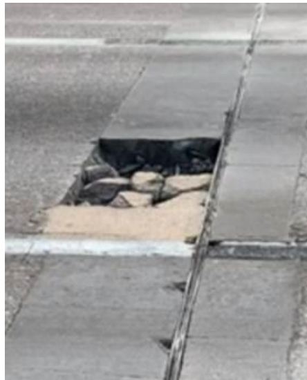
Figure 3: Failed patching materials on bridge deck on I-77 causing large potholes
