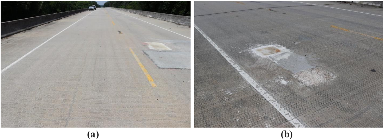
Figure B-8: (a) Pavement Surface of US 17 over Sampit River (b) Potential RSPM Incompatibility with Subsequent Repairs
