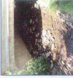
Oversized culvert with natural bottom, Route 10 over Steele Brook
