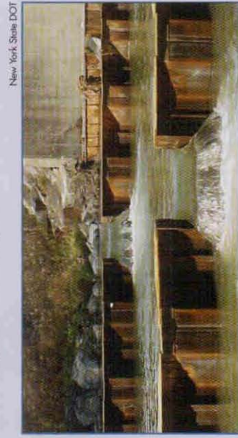
Steel overhangs on Spooner Creek fish ladders
