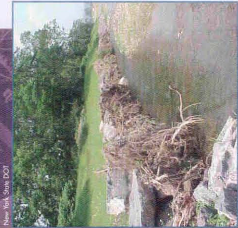
Logs and root wads help stabilize Seeley Creek
