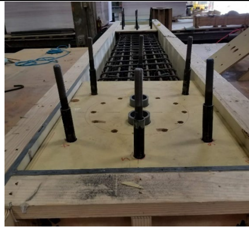
Formwork for cap-beam
