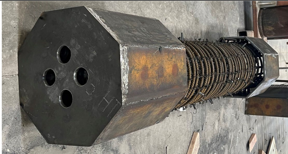
Column rebar cage with steel collar on both-sides
