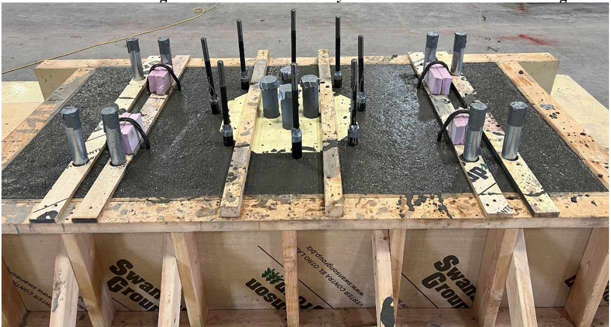
Footing after casting
