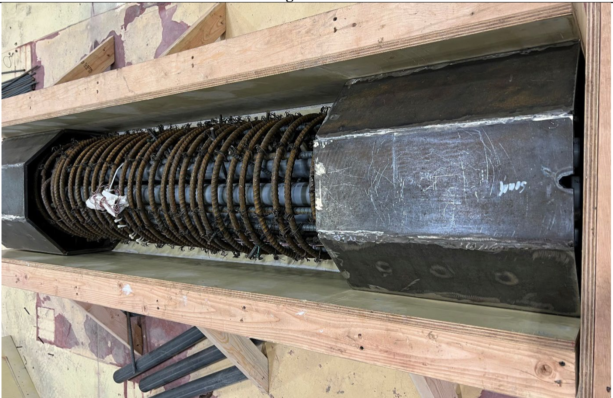
Column reinforcement inside the formwork with opening in collar
