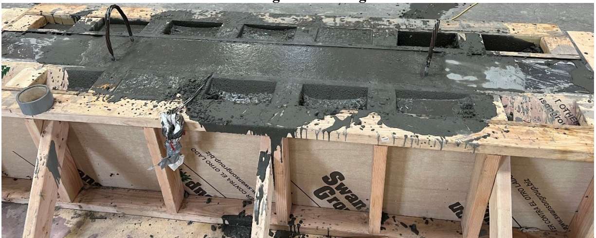
Column after casting
