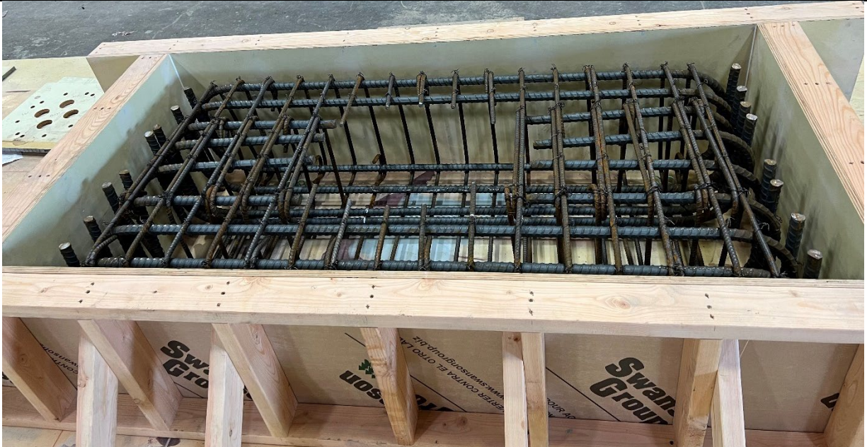
Footing steel reinforcement cage inside the formwork
