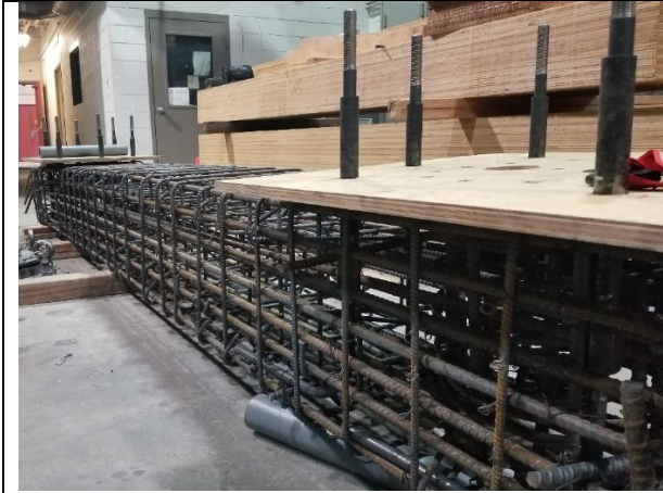
Steel reinforcing cage for cap-beam
