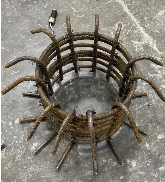
Reinforcing steel cage below shear key
