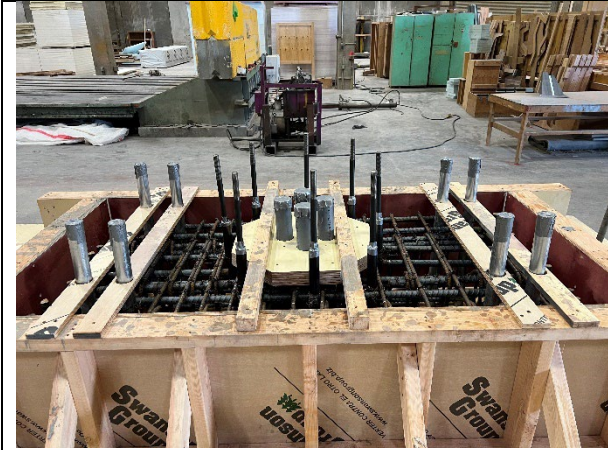
Footing rebar cage inside formwork before casting
