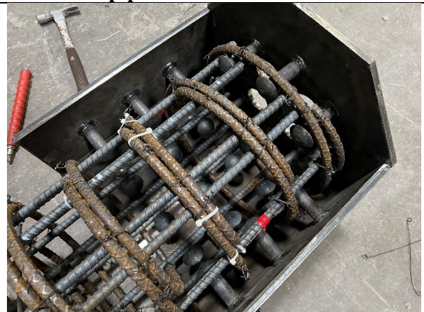
Half collar placement in column rebar cage
