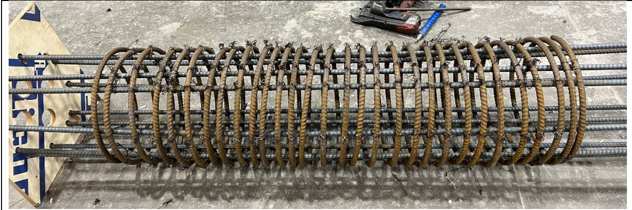
Column steel reinforcing cage
