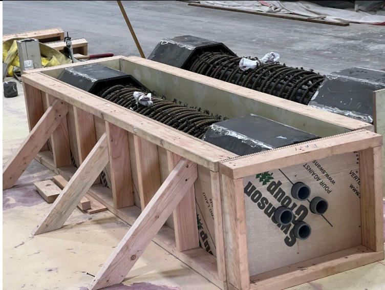
Column rebar cage inside the formwork
