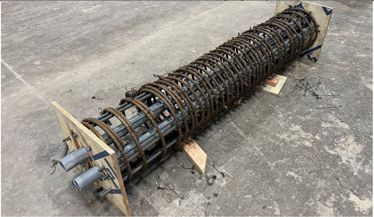
Column steel reinforcing cage with PVC pipes for PT bars
