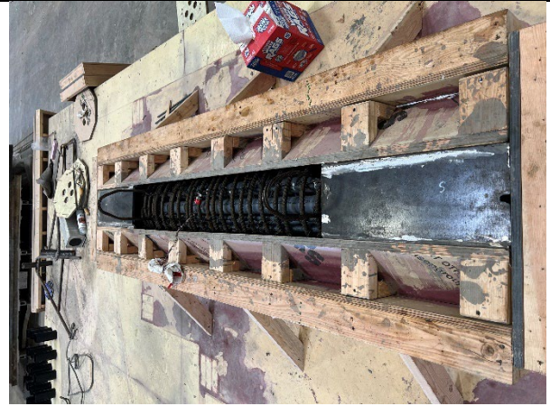
Column rebar cage inside formwork before casting
