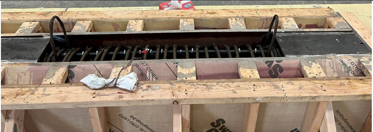
Column rebar cage inside formwork with eyes to lift the column after casting
