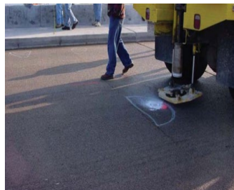
Isolated cracks and spalling in wearing surface above panel joints. Minor fiber exposure in FRP top surface. Location 5.
