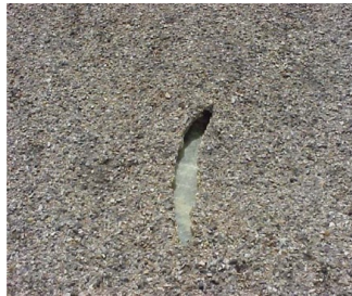
Wearing surface delamination and minor scratch. Location 1.
