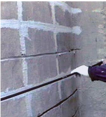
603 FRP Near Surface Mounted (NSM) Reinforcing Bars
