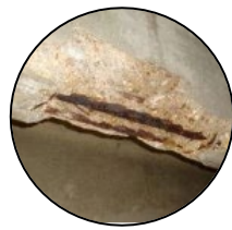
F.2 Steel Corrosion
