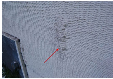
Wrinkling, 4 inches long, in GFRP sheet at crashwall of Pier 2.
