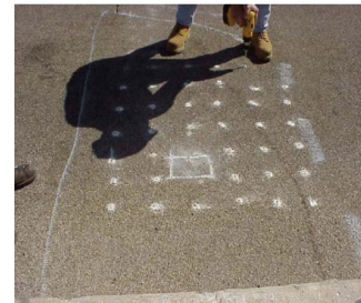
Isolated blisters, 1-inch diameter. Locations 2 and 3.
