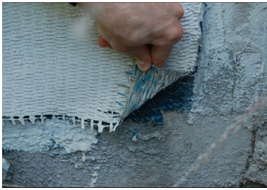
Debonding, 6-inch diameter, at the easternmost column of Pier 2.
