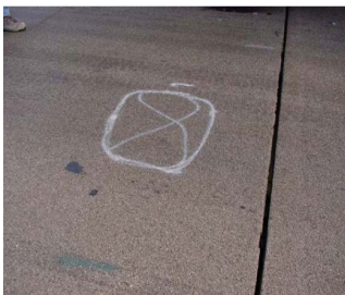
Isolated debonding, 6-inch diameter. Location 4.
