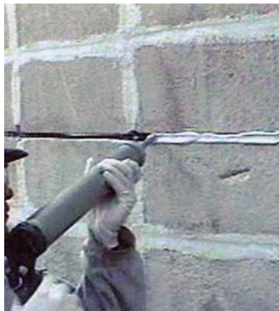
603 FRP Near Surface Mounted (NSM) Reinforcing Bars
