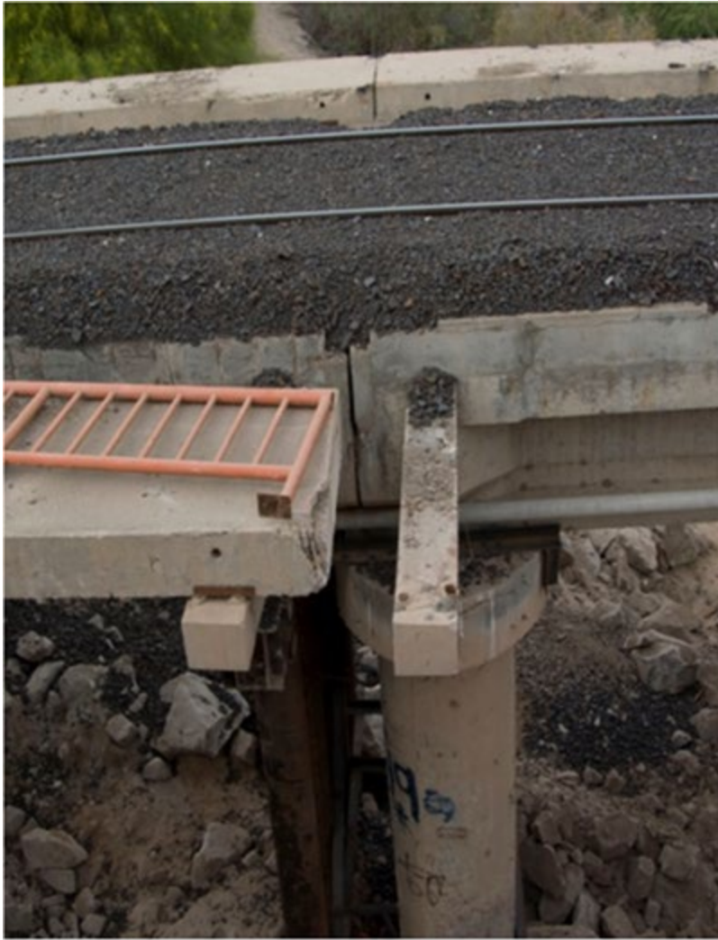
(a) Nearly unseated Span at Bent B2 of Railroad bridge
