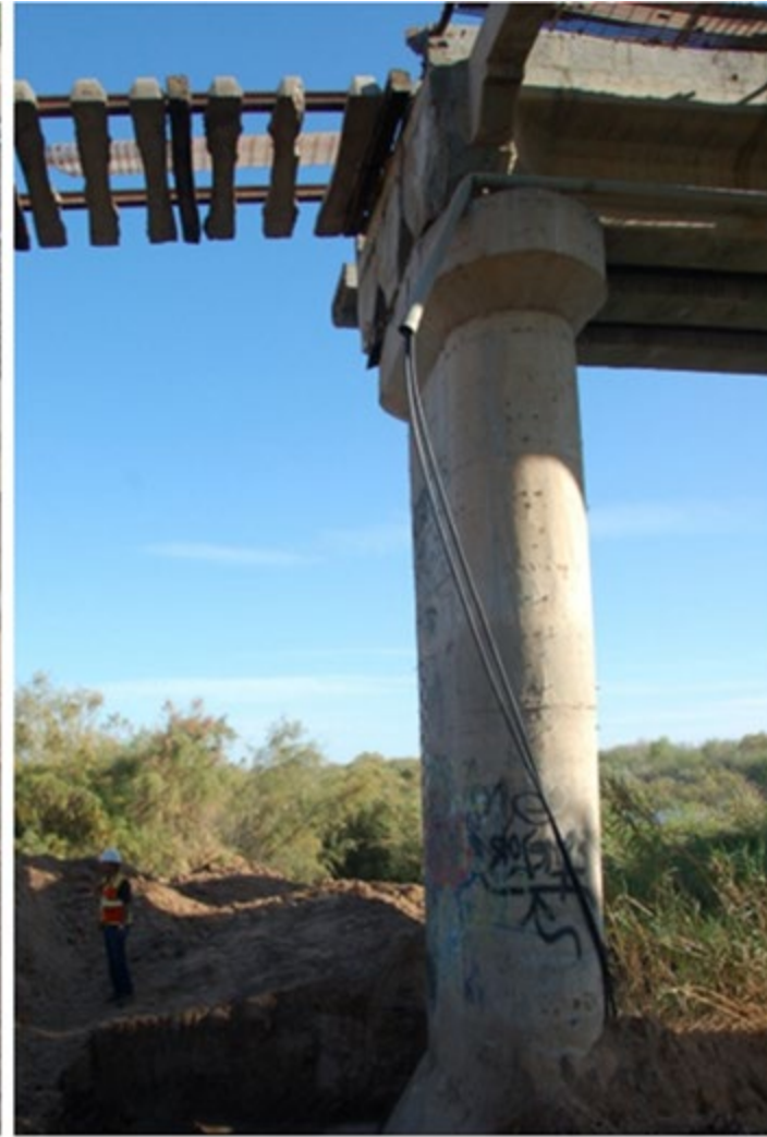
(b) Unseated Span at Bent B5 of Railroad bridge
