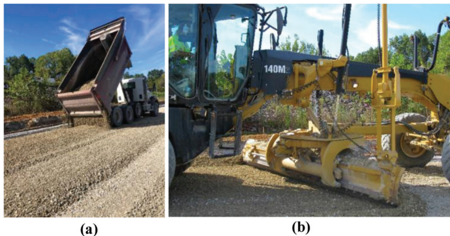
Figure 4.11 Construction stages at Site 2: (a) placement, and (b) spreading and leveling of aggregate.
