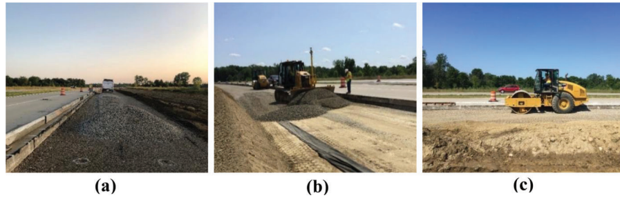
Figure 4.2 Construction stages at Site 1: (a) placement, (b) spreading and leveling, and (c) compaction of aggregate.
