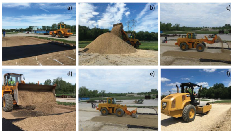
Figure 3.4 (a) Methods used for the construction of aggregate layers and the placement of geotextile and equipment (note: stakes used for marking testing grid), (b) mixing, (c–d) placement, (e) leveling, and (f) compaction of aggregate.
