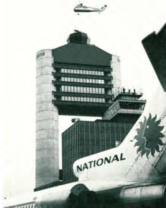
AERIAL CRANE —Quicker and cheaper than a crane, a helicopter, picked up the 2,000-pound ground control antenna from the old nine-story Logan International Airport Tower and set it atop Boston's new 22-story tower, which is scheduled to be commissioned next month.
