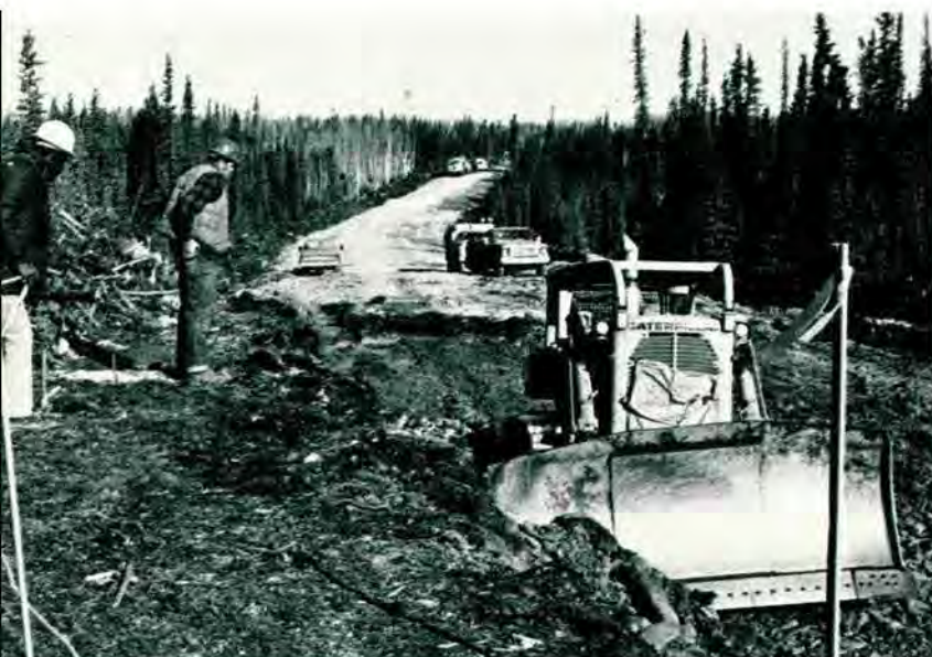
A northern section of the 360-mile pipeline service road takes shape. It will link up with existing roads south of the Yukon.
