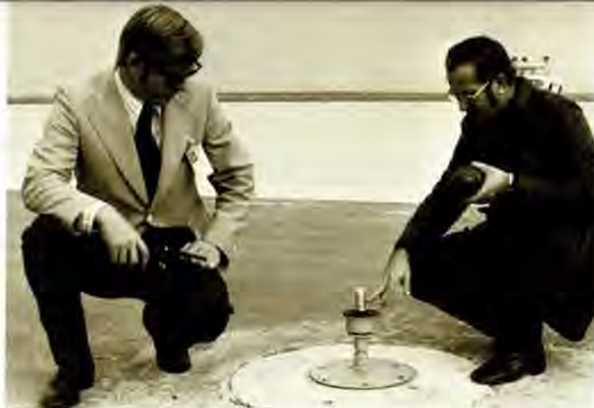
Inspector Staley (right) removes the globe to demonstrate the proper bulb alignment in a non-glare runway light to airport operations supervisor Ron Bowling.
