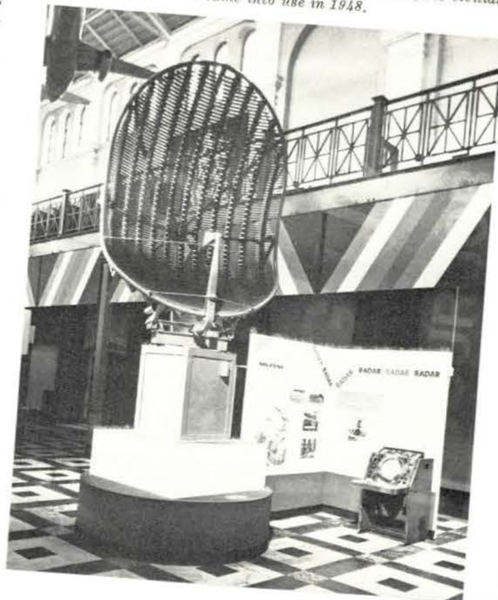
The ASR-1 radar and antenna that was CAA's first civilian radar equipment. It came into use in 1948.
