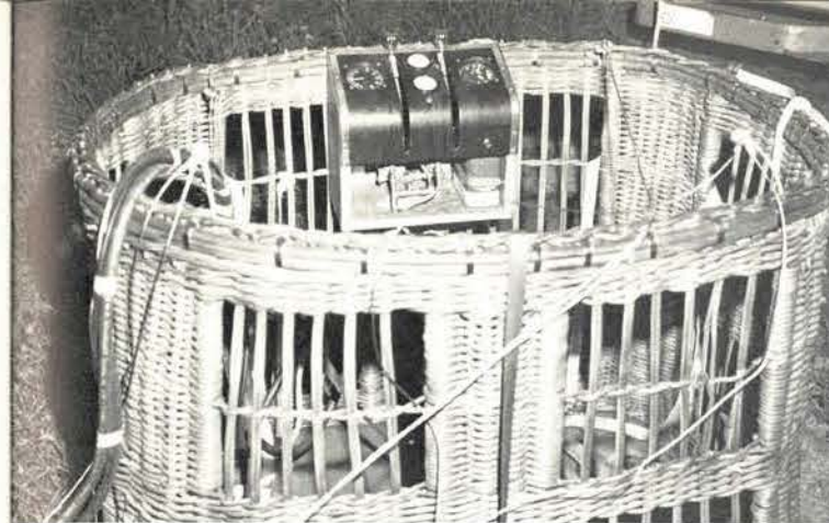
There's standing room only in the balloon gondola with the instruments for altitude, rate of climb, controls for regulating the hot air fuel and two 10-gallon tanks.
