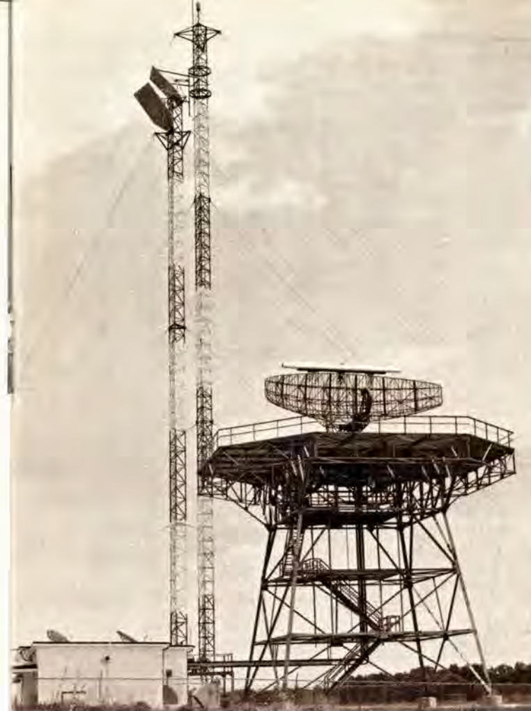
It takes lots of antennas to make a system. Shown here are the radar antenna, the beacon antenna (the bar atop the oblong radar antenna) and the microwave-link and communications antennas (the tall towers).
