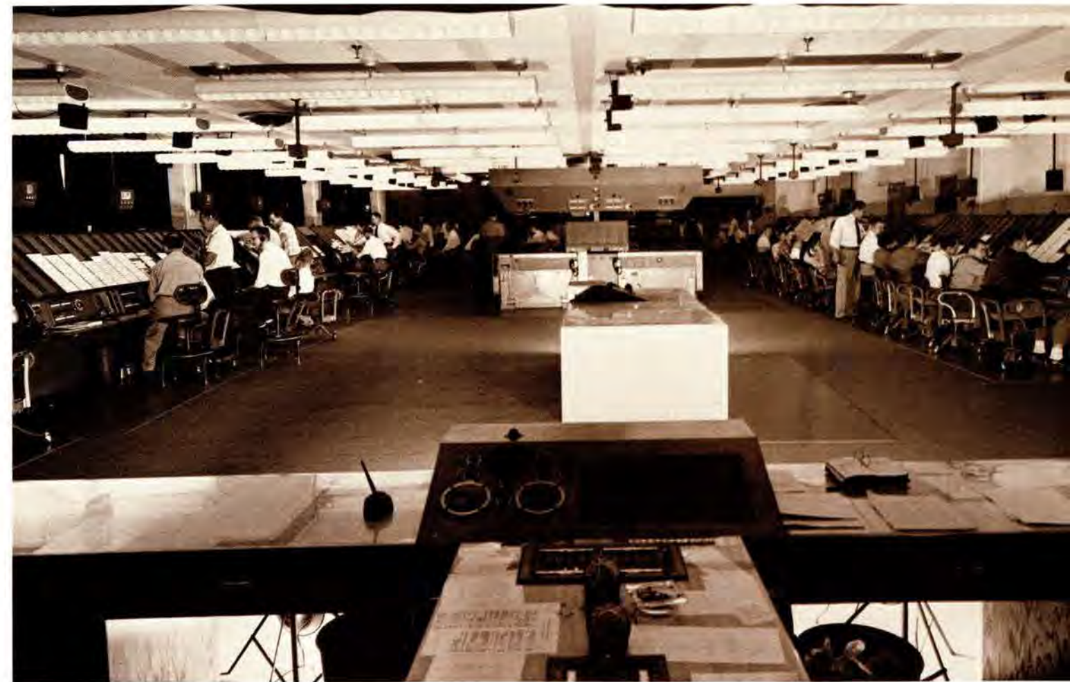
In 1955, a military radar (light-colored cabinets) was installed at the New York ARTCC, but controllers did not rely on the long-range radars until the ASR-1 program got underway.
