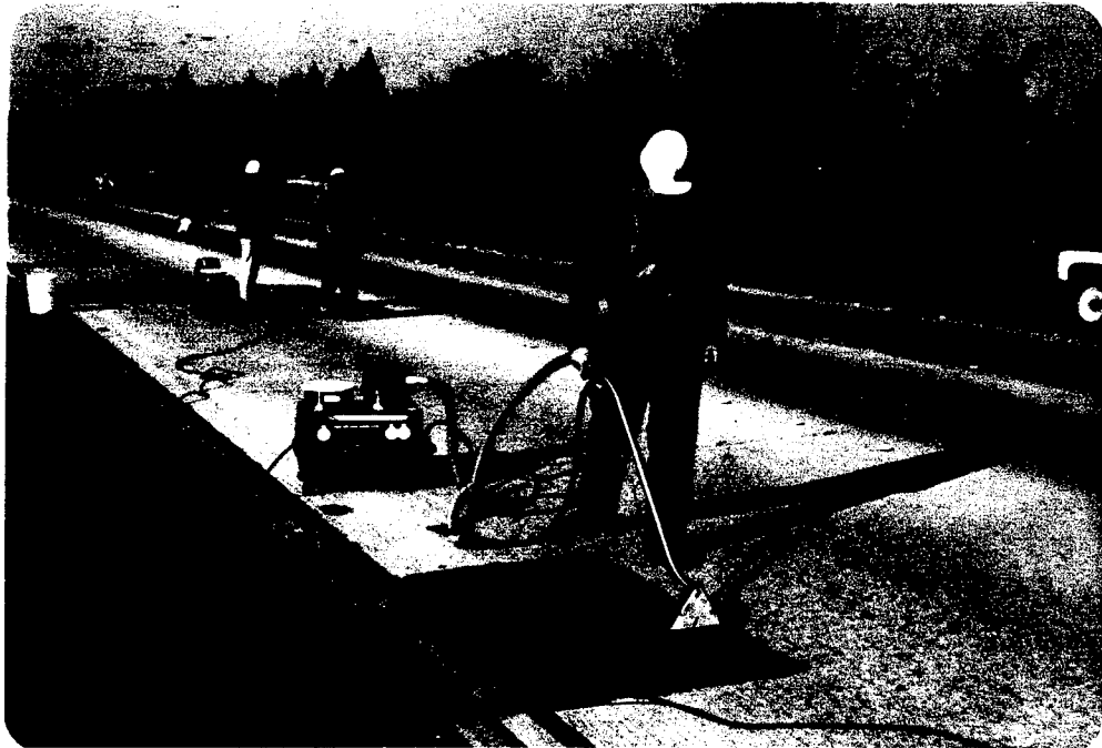
Figure 31. Flushing the highway surface.
