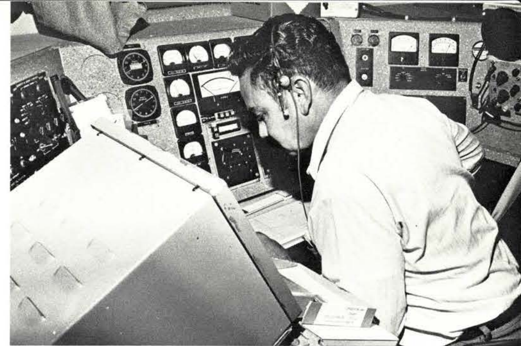
Electronic technician Thomas W. Pennington's office in the DC-3 is right behind the flight deck. His instrument console keeps tabs on the accuracy of ILS and nav aid equipment being checked.
