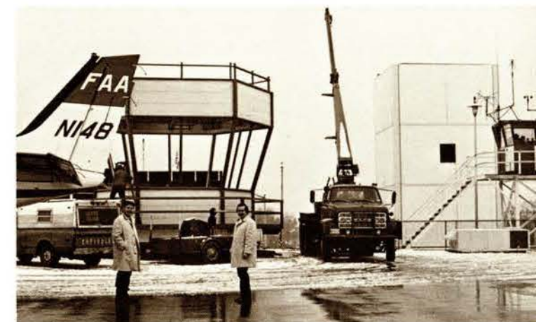
Bob Pumphrey (left), AF tower program manager, and civil engineer Jose Roman wait for workmen to rig the Morgantown, W. Va., cab for setting atop the tower shaft, in front of which is the temporary tower.
