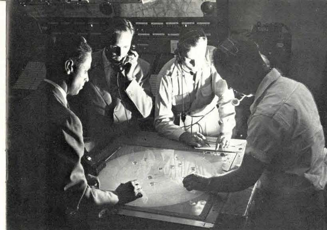
Center controllers sitting around an early long-range radar display keep track of planes by moving plastic "shrimp boats" on the display screen.
