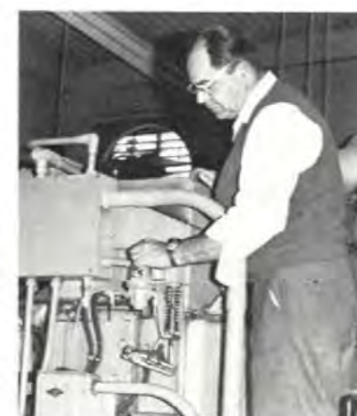
General facilities equipment technician Ed Miller inspects the fuel solenoid on the engine generator which supplies center with electricity in case of a commercial power failure.
