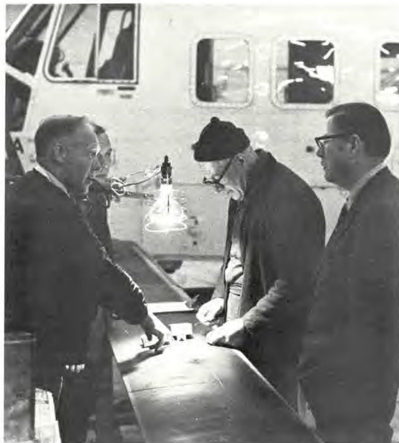
Richard Blenheim, lead mechanic for New York Airways, reinforces giant rotor blade for Sikorsky S-61L helicopter, as air-carrier-maintenance SWAP-team inspector Dick Dodd (right) observes. Showing Dodd the process are Bob Mitchell (left), company quality-control supervisor, and Martin Conway, director of technical services.
